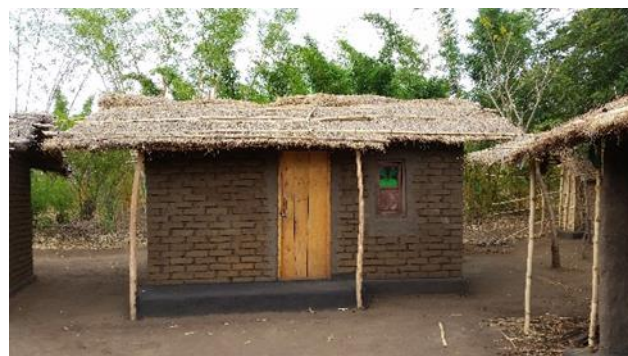
Figure 7 Typical rural homestead structure
