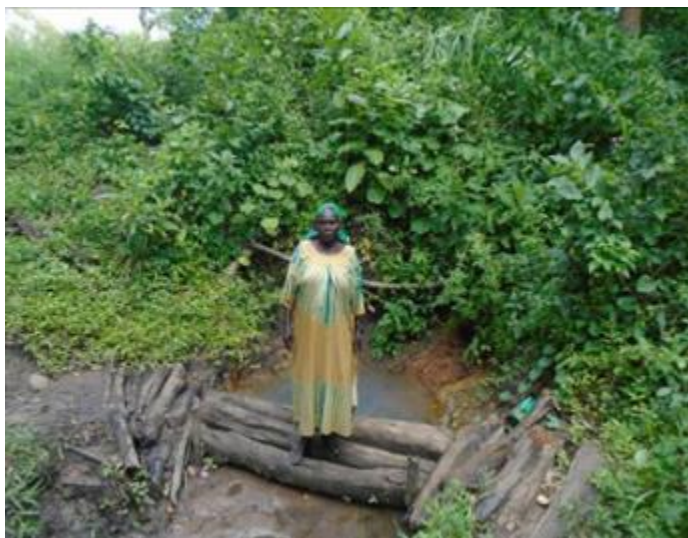
Figure 8-20 Unprotected well in Agonga A, Nwoya District
