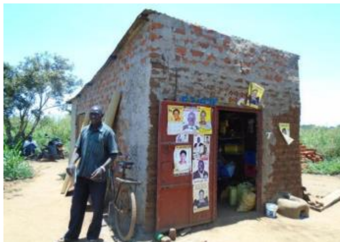
Figure 8-10 Commercial structure in Tochi, Gulu District
