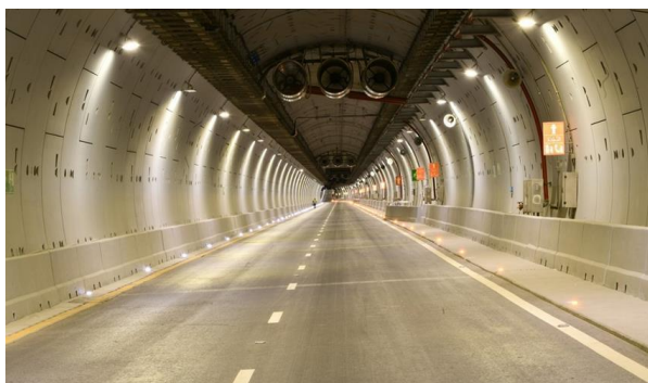
Illustration 137 3rd of July Tunnels (Port Said Tunnel)
