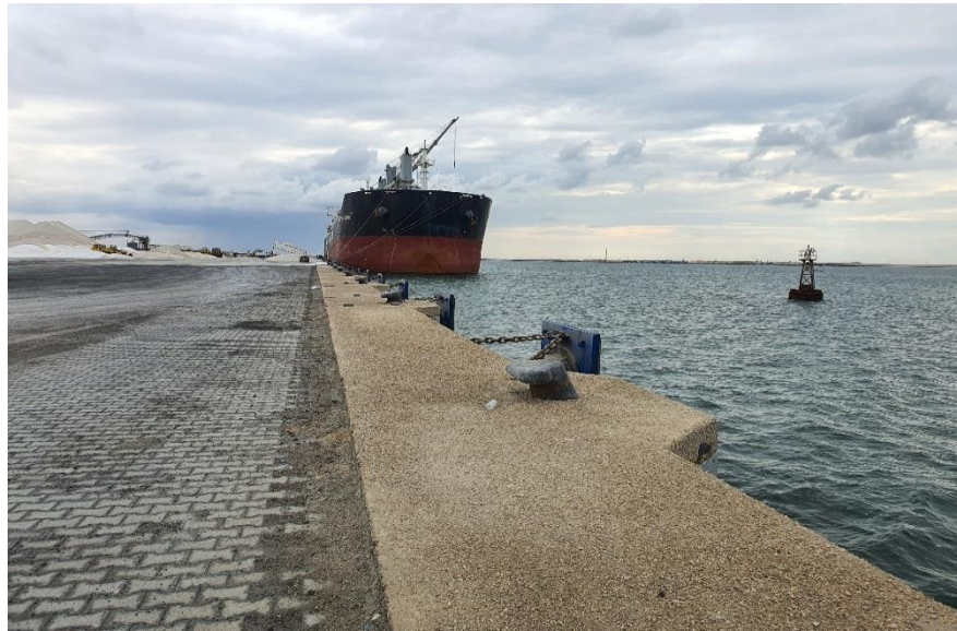
illustration 11 Columns and fenders for docking
