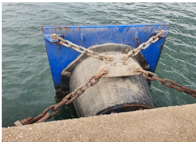
Illustration 9 Naval fenders for docking
