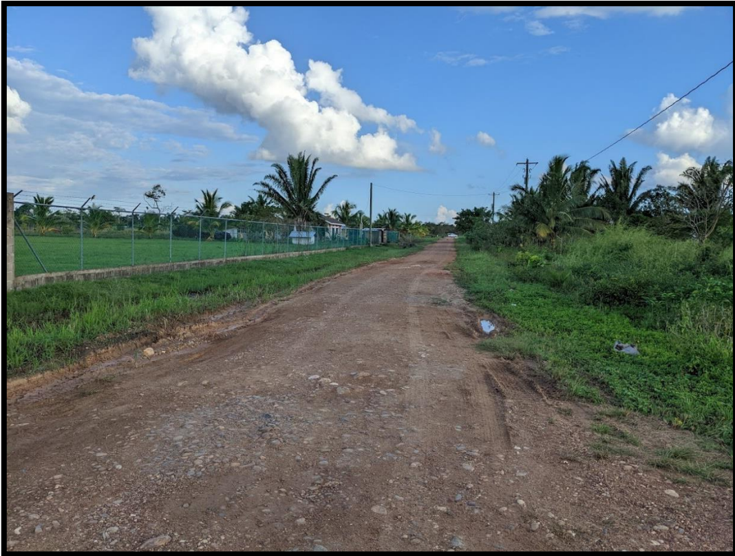
Figure 32 - Suburban profile in central proposed main in Harmonyville (Photo: PlanEHS, Nov. 2022)
