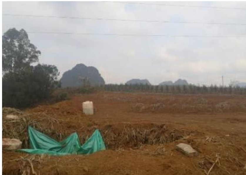
Figure A1-1: Water Supply Project (Phase 1) under construction
