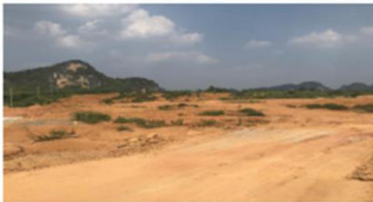
North of the project
