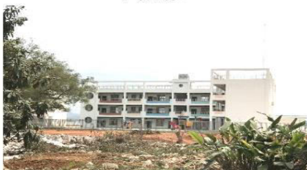
No.2 Elementary School in Xinhe Township ←
