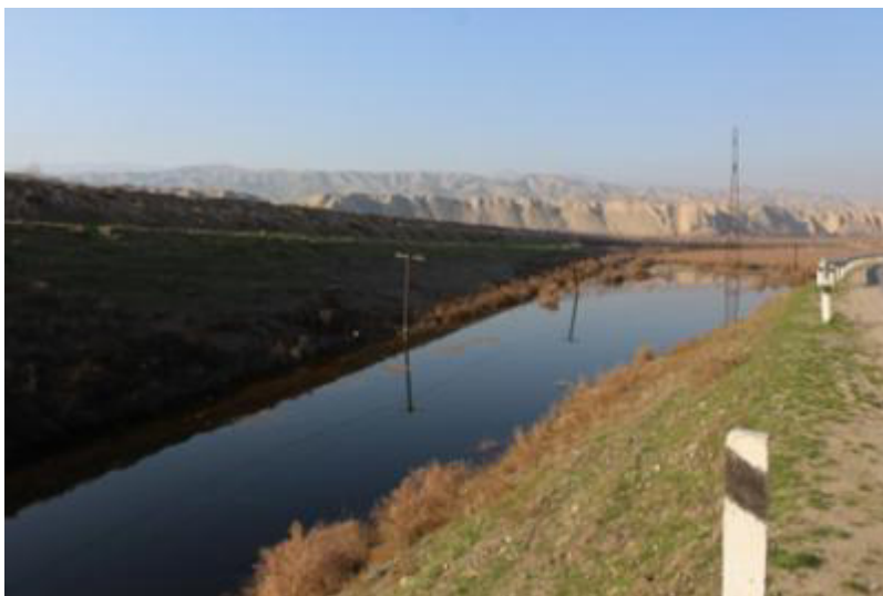
Fig. 17: Waterlogged area alongside Project road at km 66+000 – 67+500
