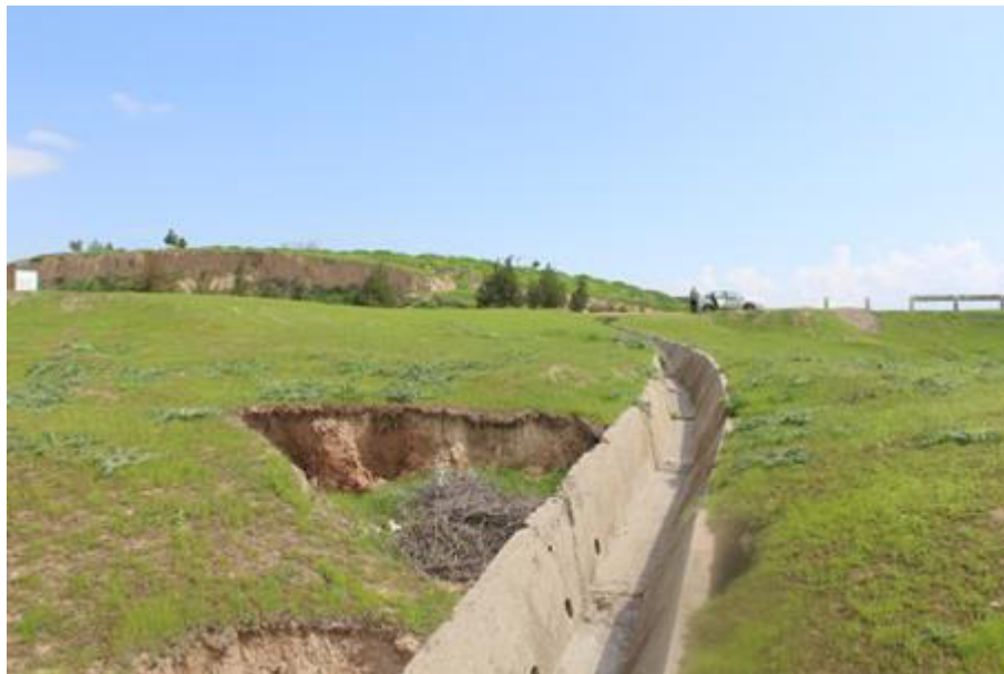
Fig. 16: Rests of a former drainage channel
