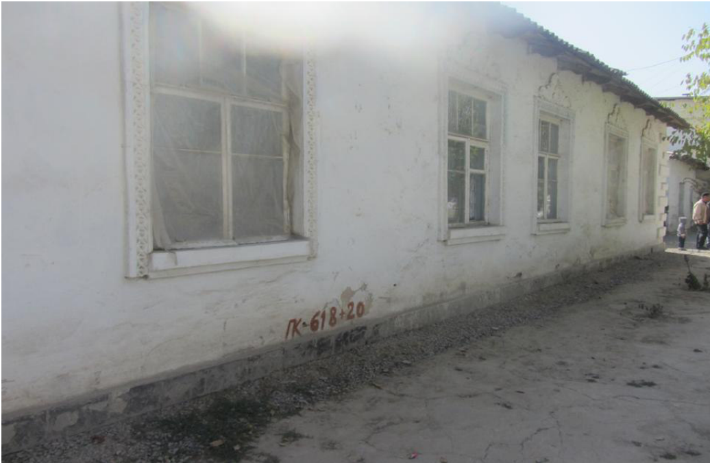
Fig. 38: Typical fairly old house alongside the project road (Km 61+810 to Km 61+835). Construction material is made of clay brick masonry.
