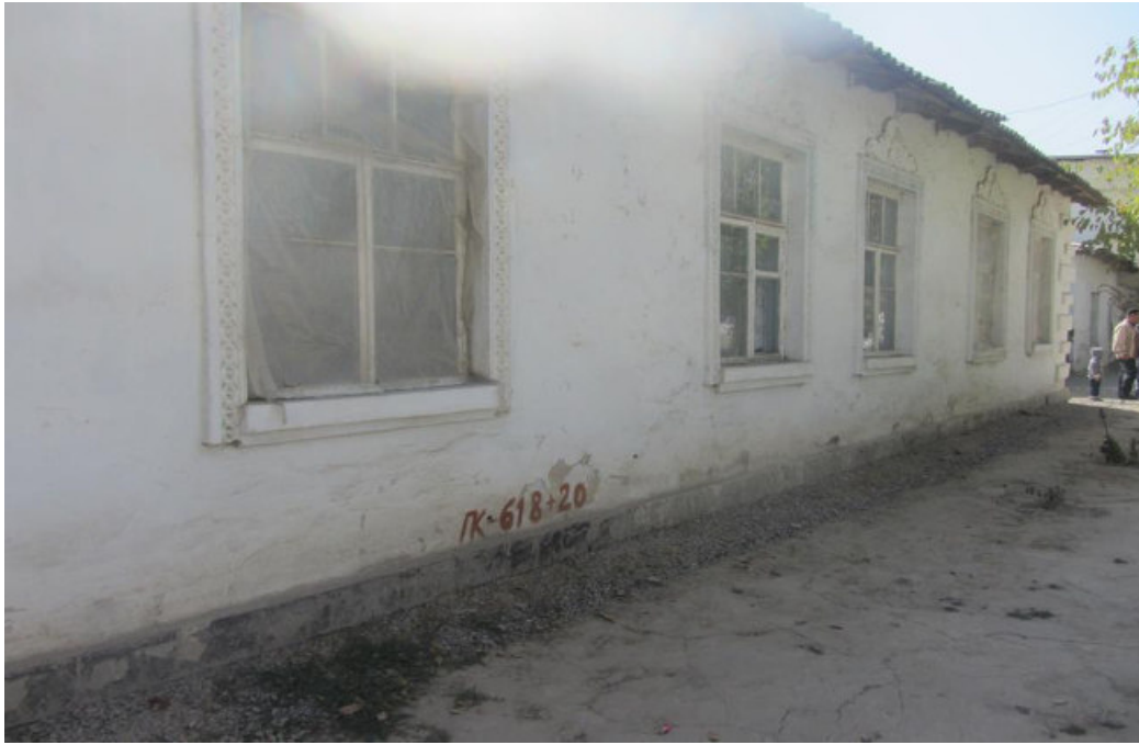
Fig. 38: Typical fairly old house alongside the project road (Km 61+810 to Km 61+835). Construction material is made of clay brick masonry.
