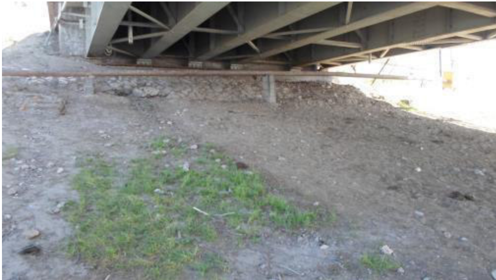
Fig. 35: Embankment of Vaksh River Bridge
