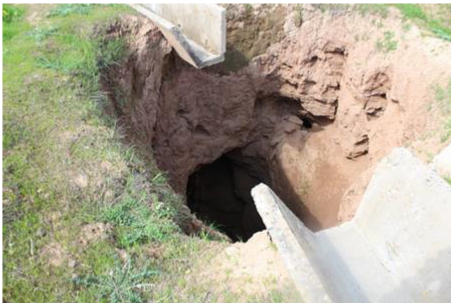
Fig. 15: The deep cave in loess-like sediments washed due to failure of drainage
