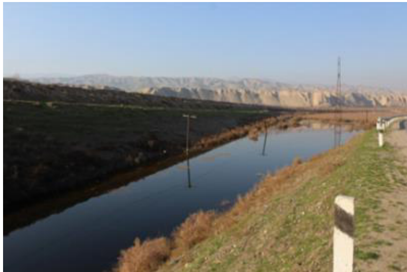
Fig. 17: Waterlogged area alongside Project road at km 66+000 – 67+500
