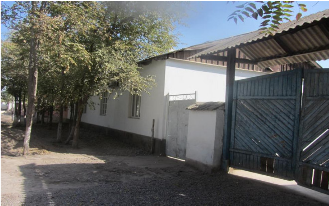
Fig. 37: Typical new house alongside the project road (Km 61+770 to Km 61+805). Construction material is made of clay brick masonry.
