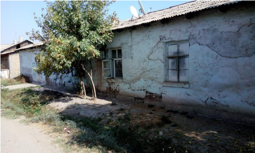
Fig. 36: Typical old house alongside the project road (Km 62+065 to Km 62+095 Left Side). Construction material is made of burnt bricks.
