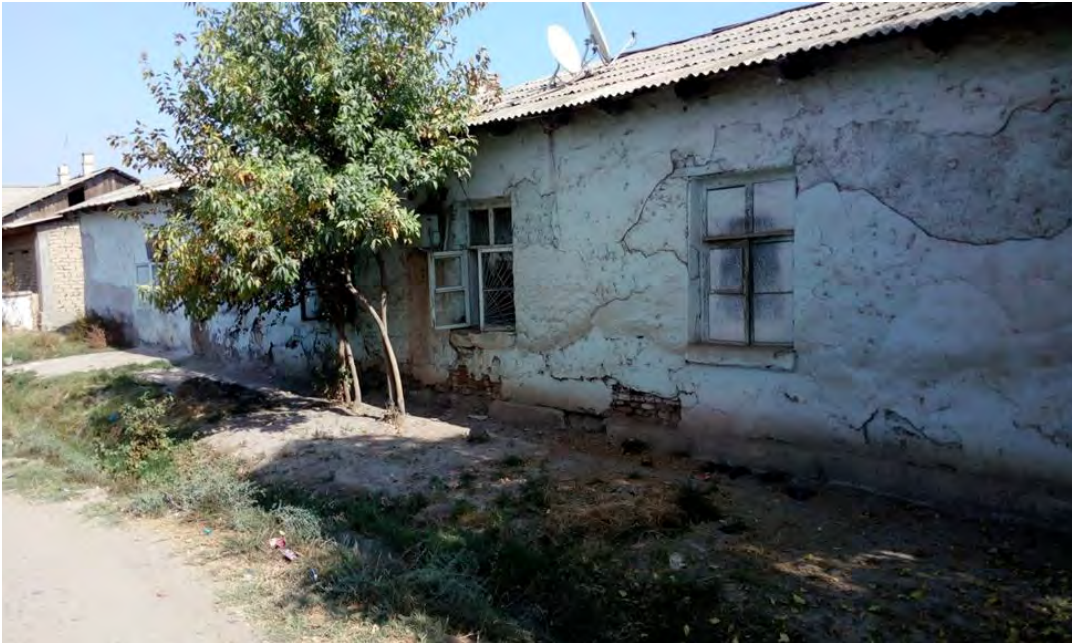
Fig. 36: Typical old house alongside the project road (Km 62+065 to Km 62+095 Left Side). Constrution material is made of burnt bricks.
