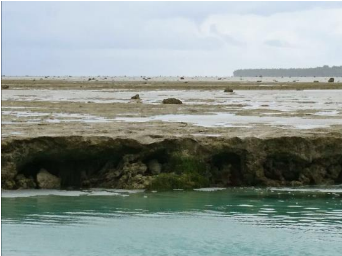
Plate 4.1: Large voids below the reef platform
