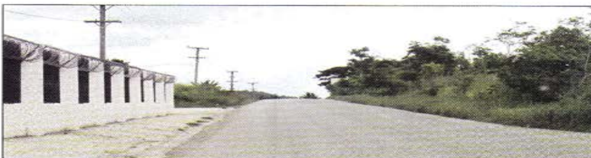
An example of encroaching onto the road reserve, which is against this new Act.
