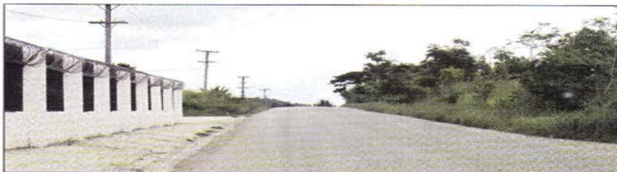
An example of encroaching onto the road reserve, which is against this new Act.
