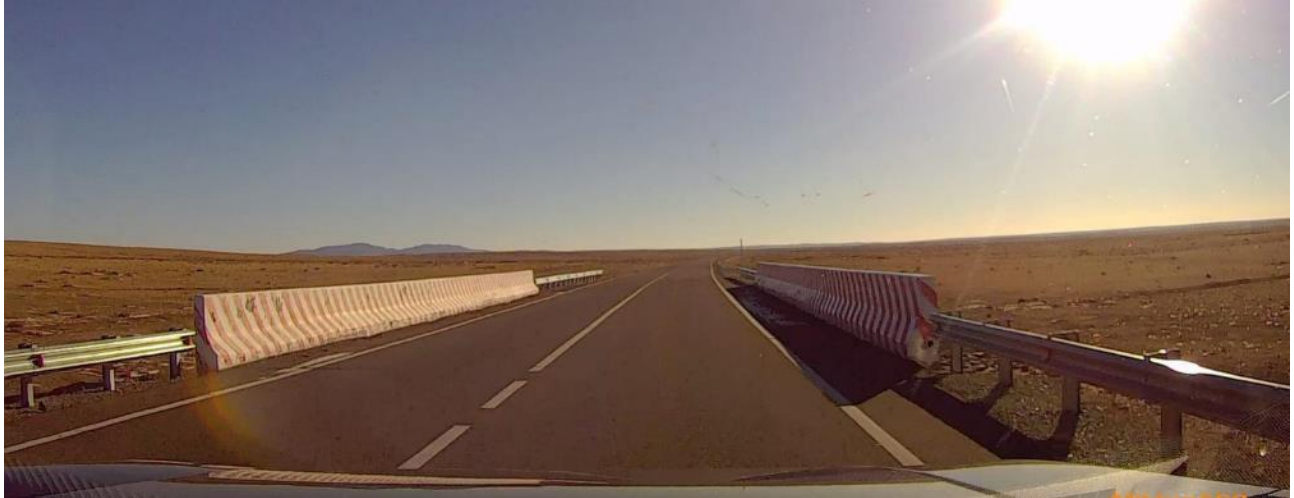
Figure III-8: Guardrail Not Connected to Bridge Abutments
