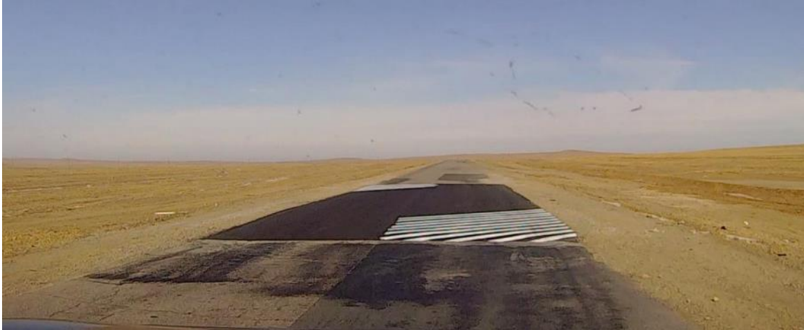
Figure III-4: Patch that Is Not at Correct Level
