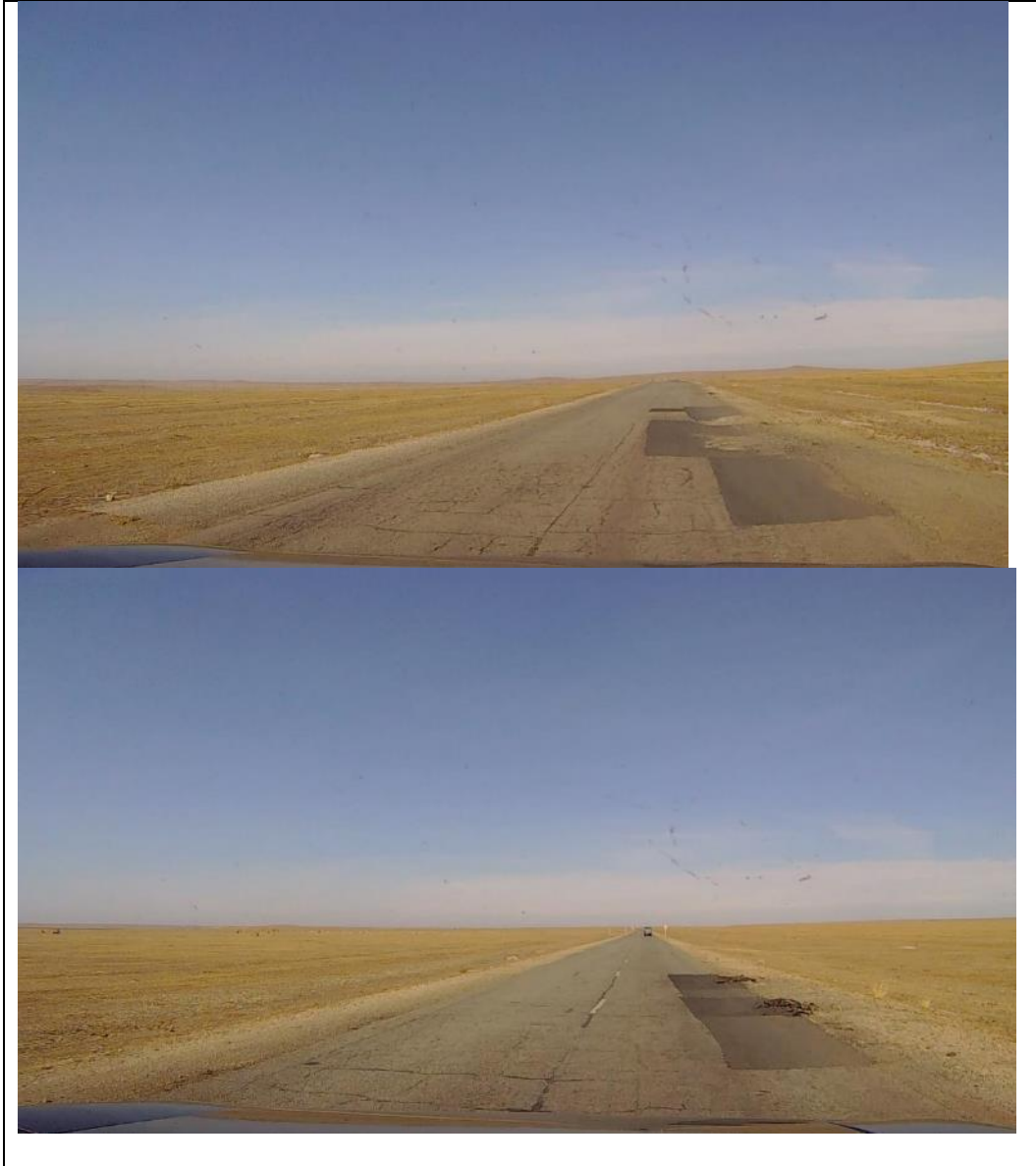
Figure III-3: Examples of Failed Minor Repairs
