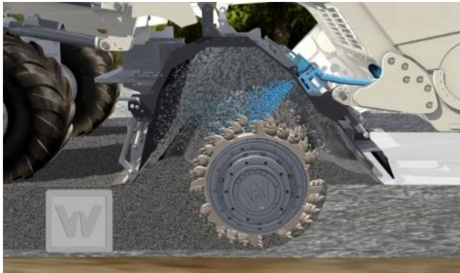
Figure 6. Sample image of In-situ stabilization process
