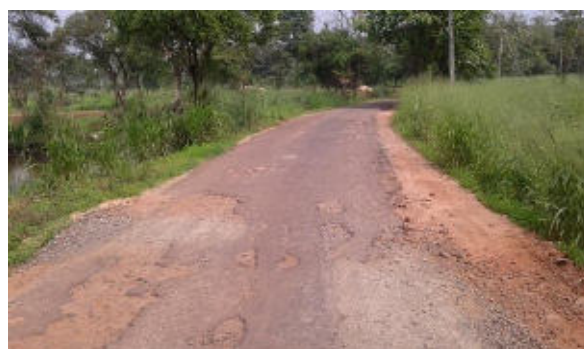
Figure 11: Damaged access road needing repair
