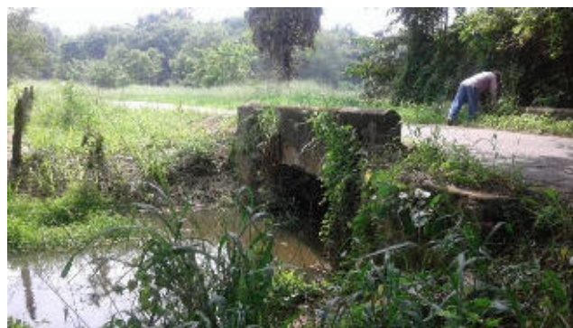
Figure 12: Culvert requiring rebuild at 3.3 km
