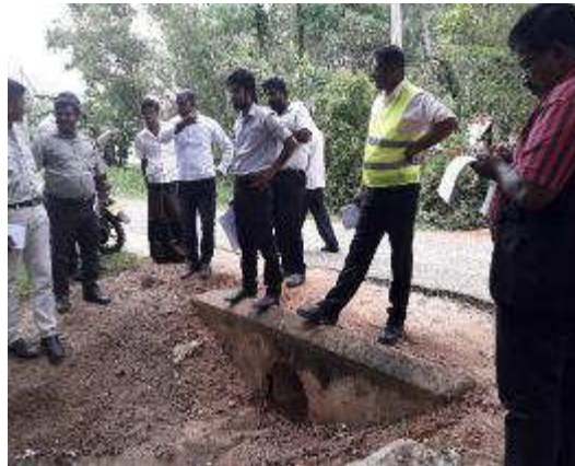
Fig.32 Blocking Culverts create lead away issue
