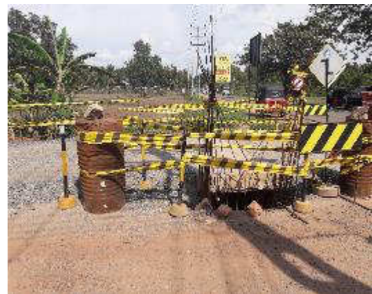
Fig.79 the culvert partly constructed without a lead away at Rd 40, PU-03
