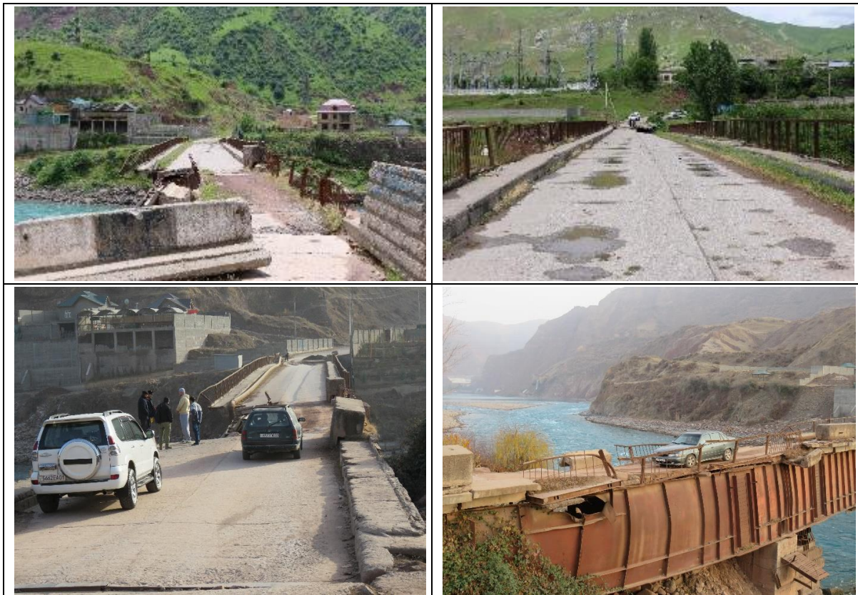
Figure 5. Current condition of bridge
