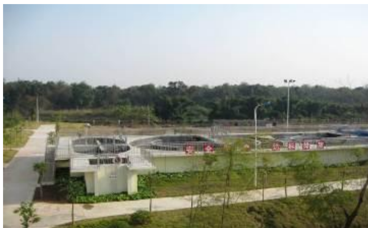
Fig. 5-3 Jingan County Household Sewage Treatment Plant
