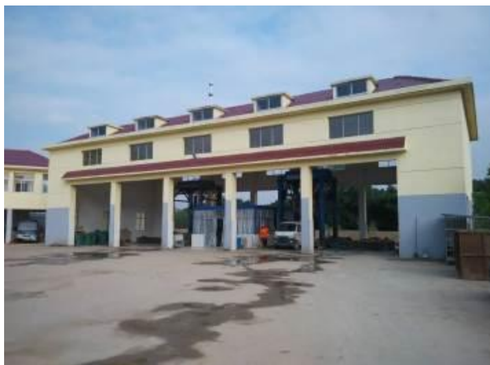
Fig. 3-2 Existing Garbage Transfer Station of Jingan County
