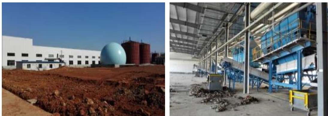
Figure 5-7 Installation and commissioning of Duchang county waste treatment plant
