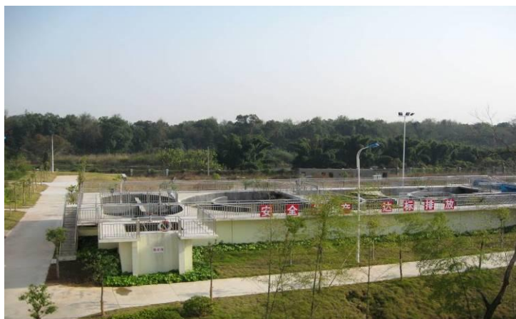
Figure 5-13 Jing'an county domestic wastewater treatment plant
