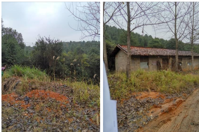
5-8 Proposed site of the MSW transfer station in Hengshui Village, Jinshan Town
