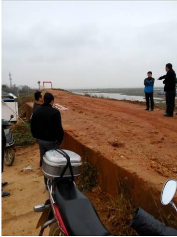
Zhuhu Lake embankment
