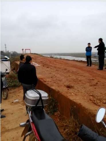
Figure 1-5 Field visit of lake embankment
