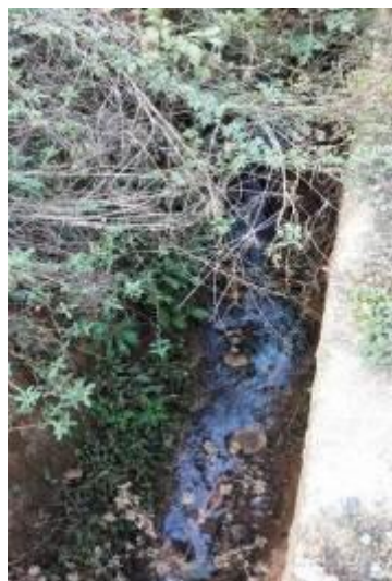
Figure 3-8 A Sewage Outlet in Furongshan Industrial Park to the West of Jinchang Road
