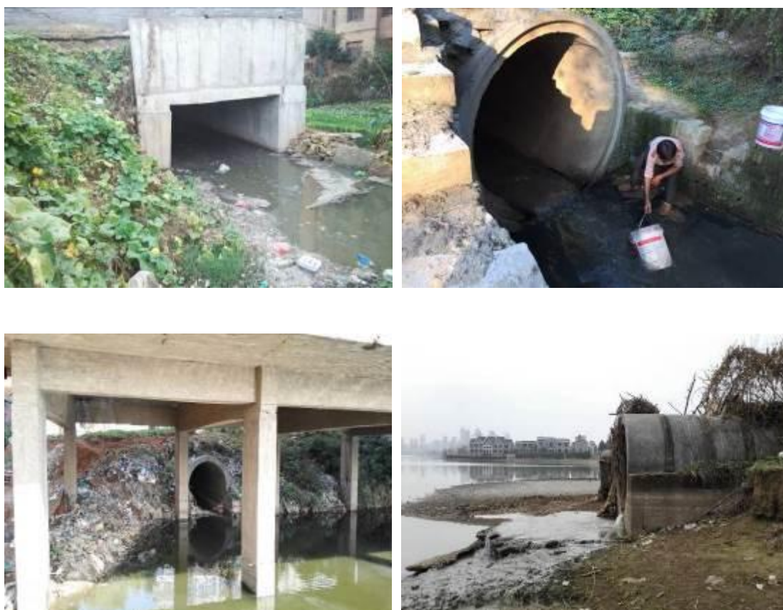
Figure 3-3 Partial Urban Sewage Outlets
