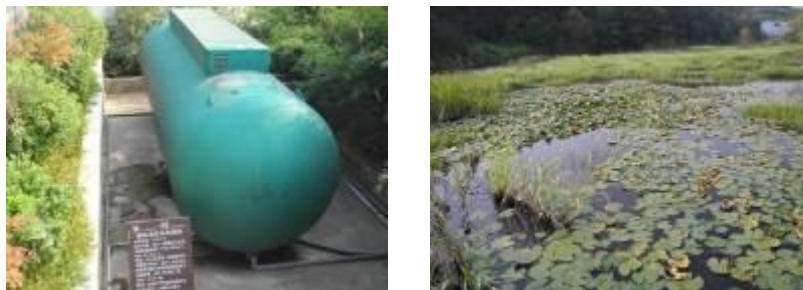
Fig. 3-6 Sewage Treatment Facility of Wetland Park Administration Committee
