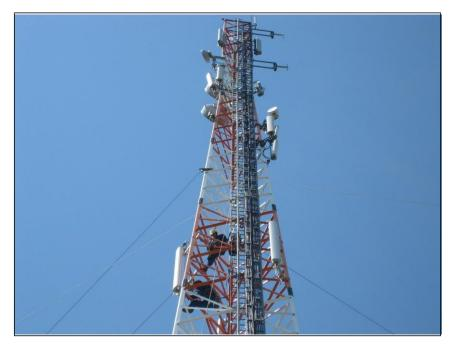
**Photo 5:** Visual Signal and Nevigational Light Installation
