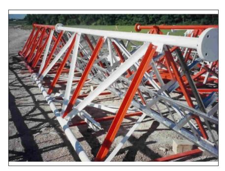
**Photo 2:** Stacking Tower Sagments at BTS Site Station
