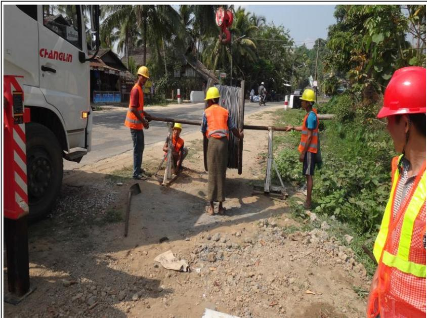
**Photo 10:** Cable Landing in Developed Land
