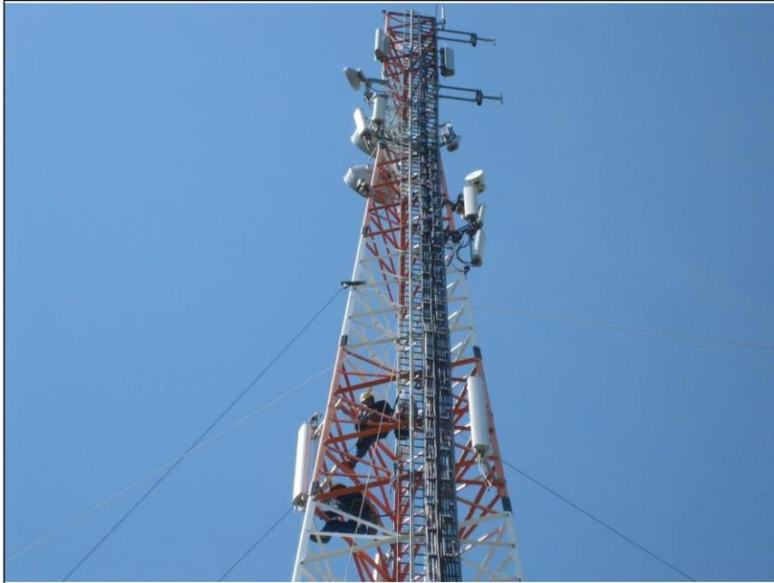
**Photo 5:** Visual Signal and Navigational Light Installation
