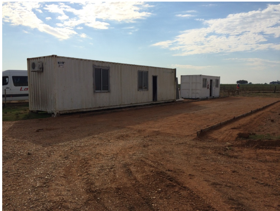
Figure 2: First office buildings installed on site
