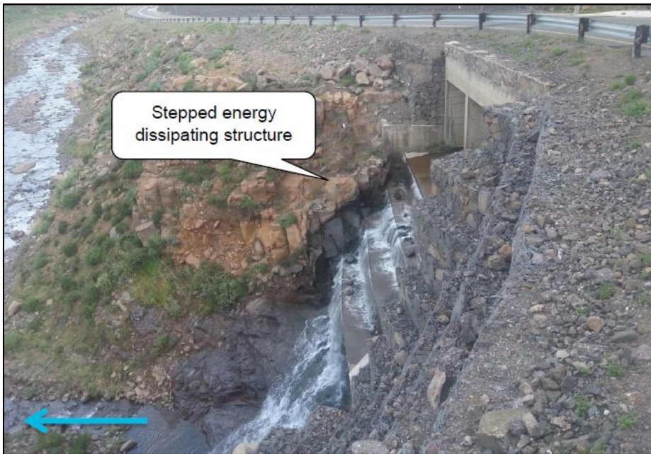
Figure 4.18 Typical Example of Stepped Energy Dissipating Structure
