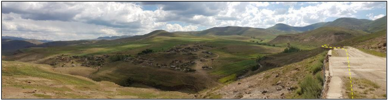
Photo 20. PWAR route along existing road kp 50
