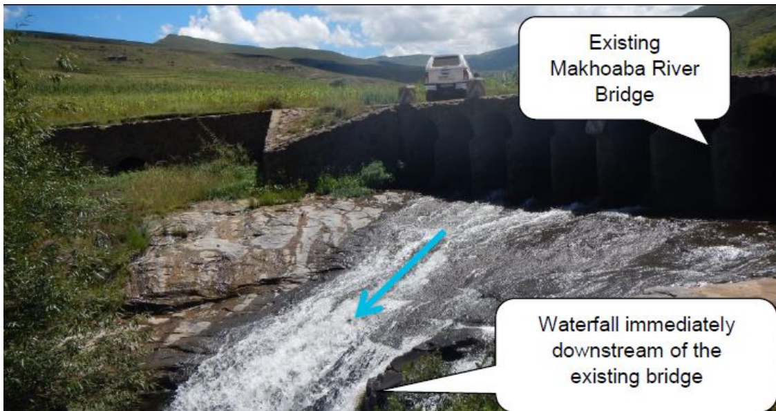
Figure 4.13 Existing Makhoaba River Bridge from the Downstream End
