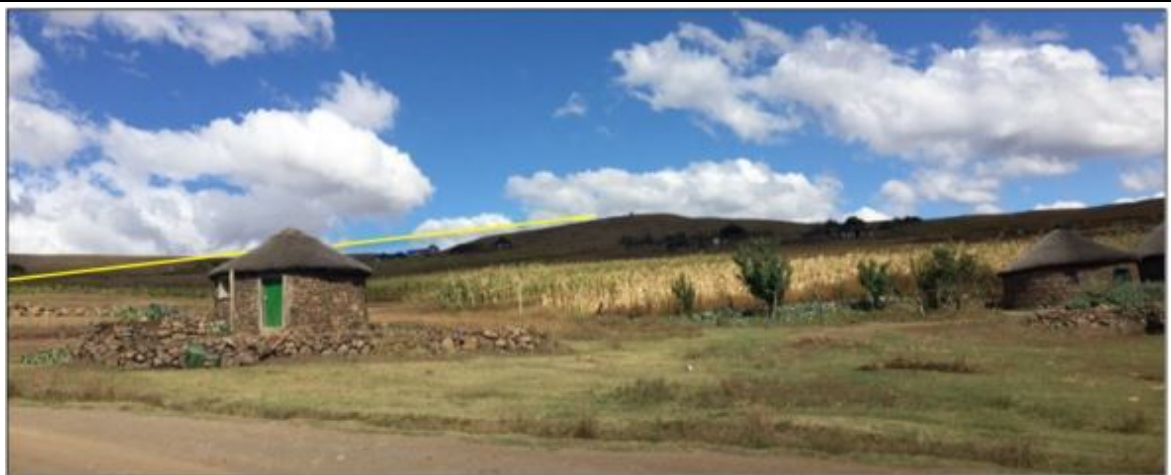
Photo Point 22: View South as TP33 crests the ridge and crosses the existing road to the Polihali substation.
