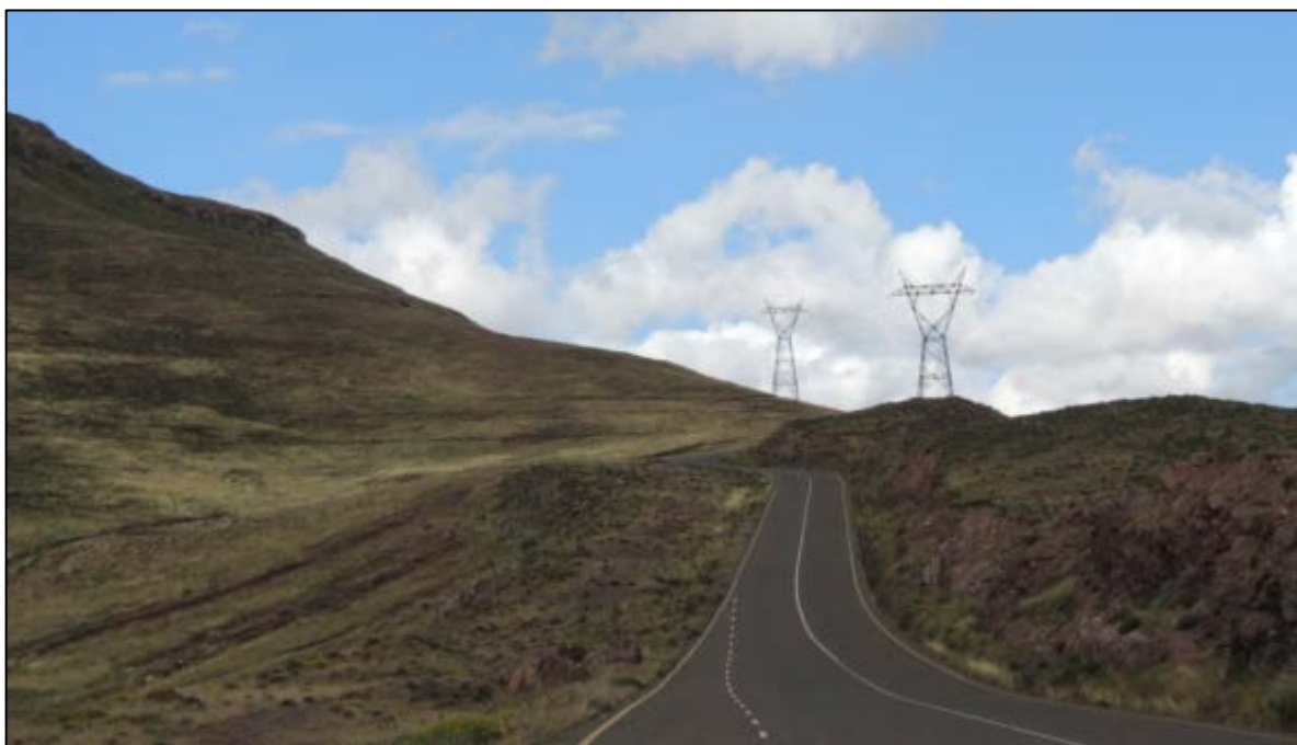
Figure 6.42 View from the A8 adjacent to Katse Dam with Pylons Located Directly Adjacent to the Road in Prominent Skyline Locations
