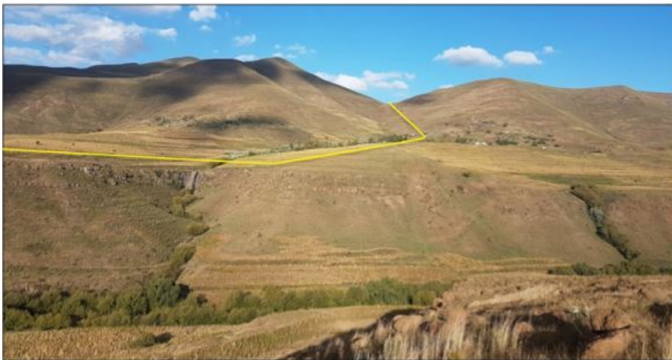
Photo Point 3: View of the powerline route across Matsoku River and up behind Ha Makhoana village at top right along bridle path (to descend the other side to Pitseng village in Liseleng valley) (pylons C4-C6).
