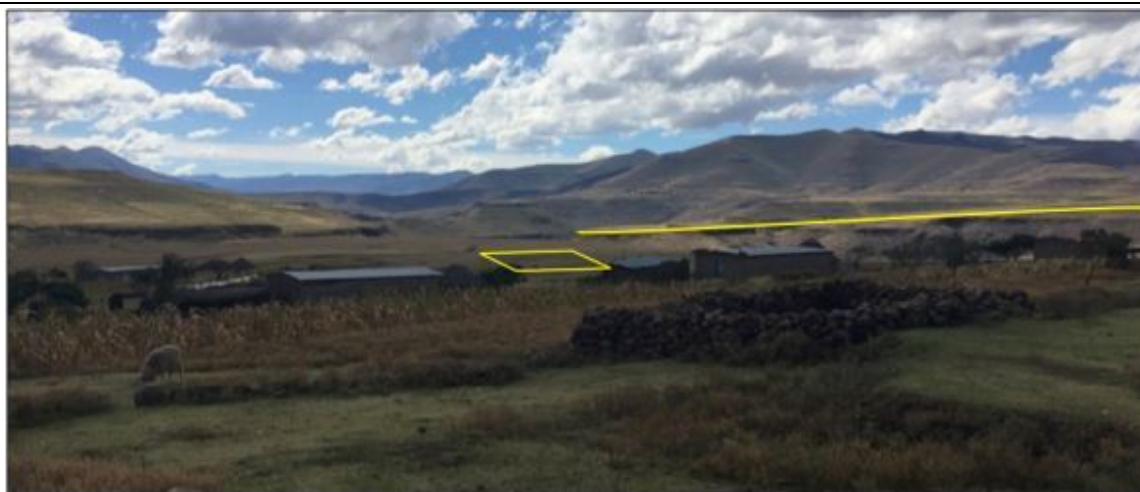
Photo Point 23: View towards the Polihali substation (approximate position).
