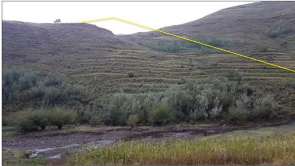
Photo Point 4: View of the Powerline as it descends from Pitseng, across the Liseleng River with poplars to join PWAR at TP 8.
