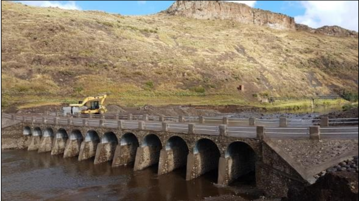
Figure 12.13 New Bridge over the Matsoku River on Route C. Note: proposed bridge on Matsoku would have three spans of 20 m width each.
