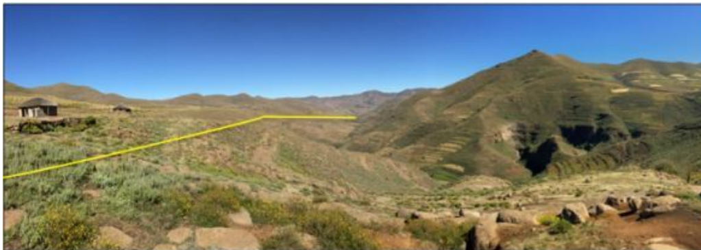
Photo Point 6: View of the Powerline Route up the Liseleng River Valley below Ha Tielase village (TP 9).
