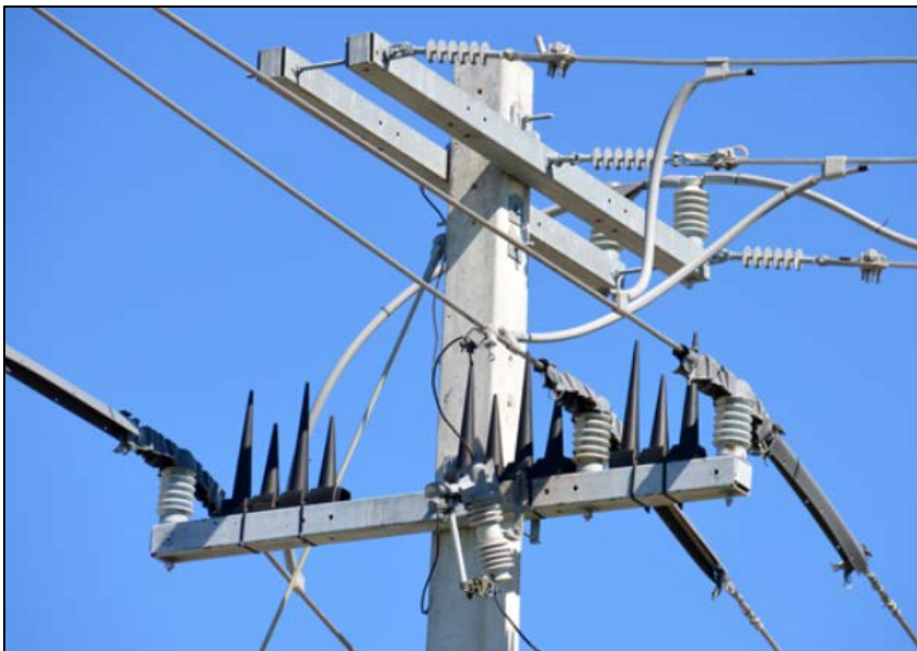
Figure 4.37 Example of Similar Bird Guard / Anti-perching Device
