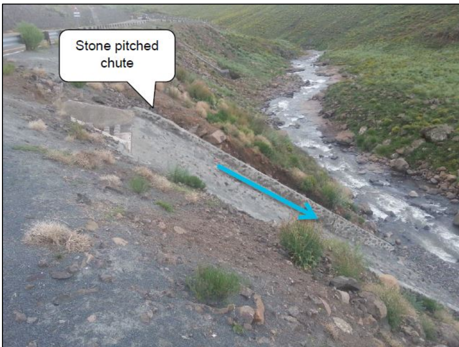
Figure 4.19 Typical Example of Major Culvert Outlet Chute
