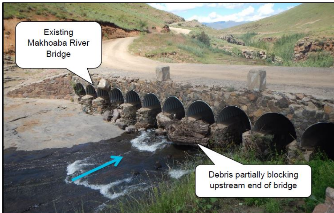
Figure 4.14 Existing Makhoaba River Bridge from the Upstream End
