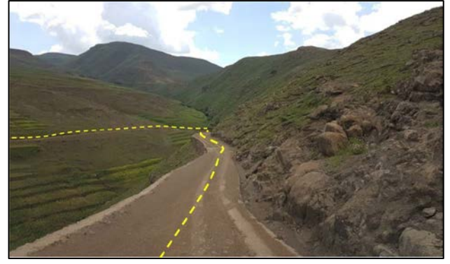
Photo 19. Well maintained dirt road from Polihali to Ha Mei (near kp 51)
