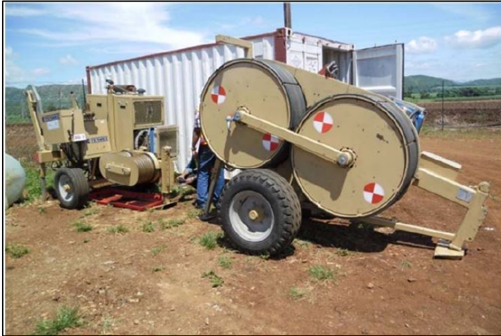
Figure 4.36 Stringset for Stringing of Powerlines
