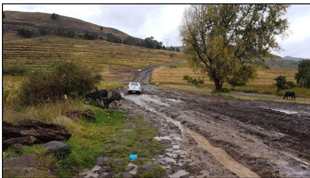
Photo 3. Existing road access from Ha Seshote to Ha Phakoeng (kp 0-1) (Note: PWAR bypasses this section)
