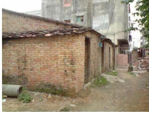
Figure 2-2 Affected Non-residential structures
