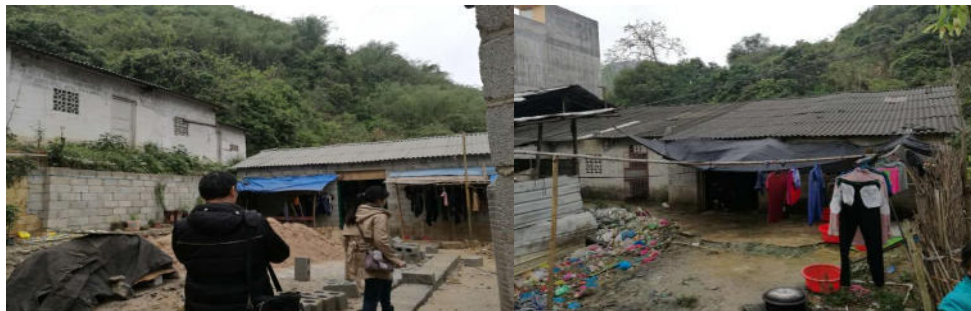
Figure 2-2: Current Status of 3 Affected Rural Houses
