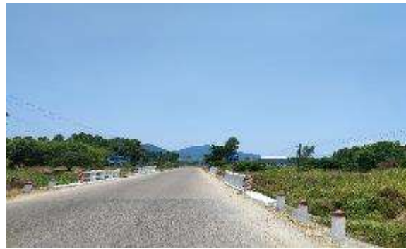
Ta Suc II Bridge
