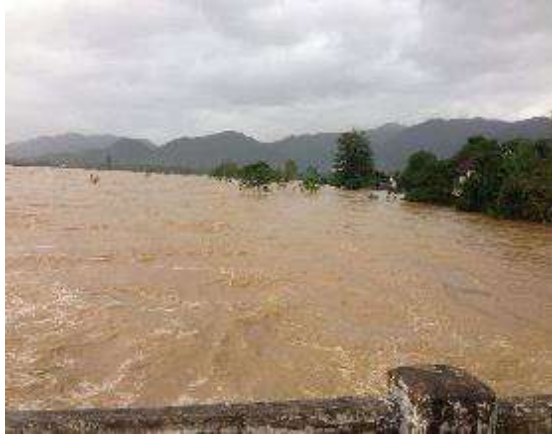
Flooding at Xem Stream Bridge
