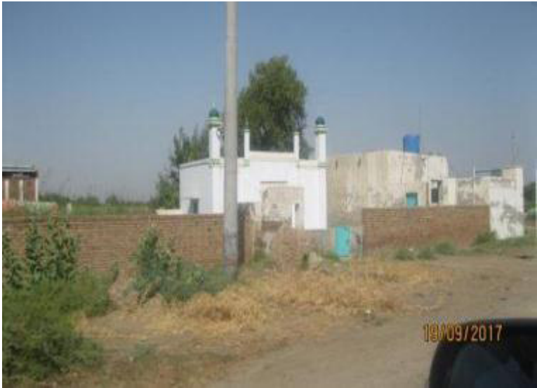
Mosque located within 30m of ROW at Kotla Nasir
