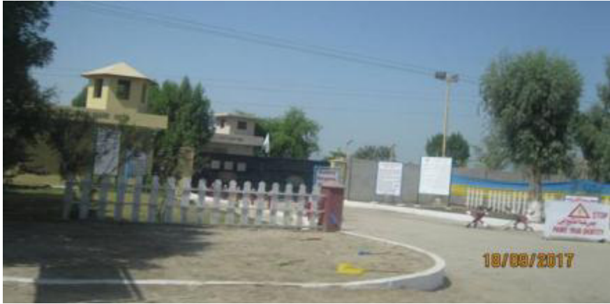
PARCO office at Faizo Laro Distt Shikarpur
