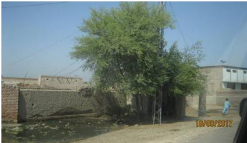
Eclectirc poles located along the road alignment
