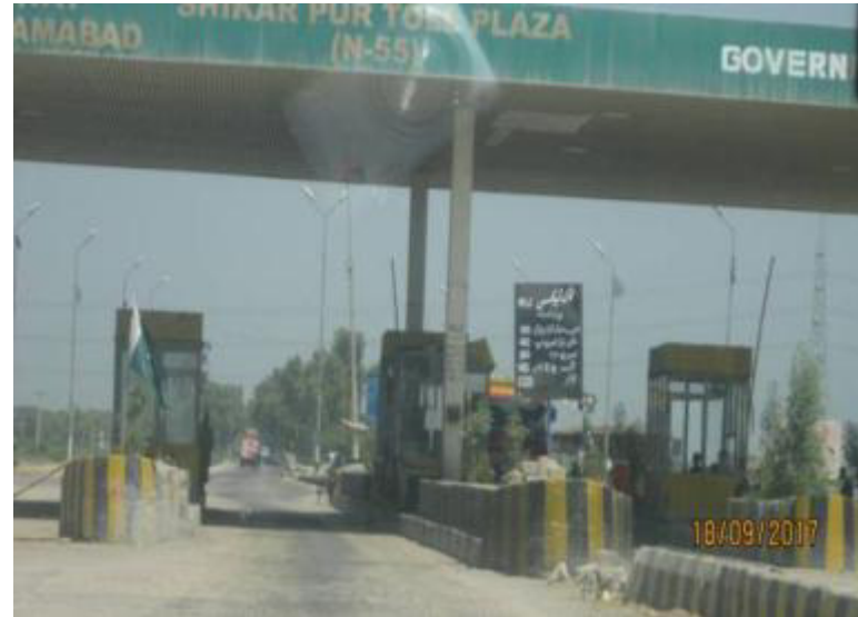
Toll Plaza, Shikar Pur
