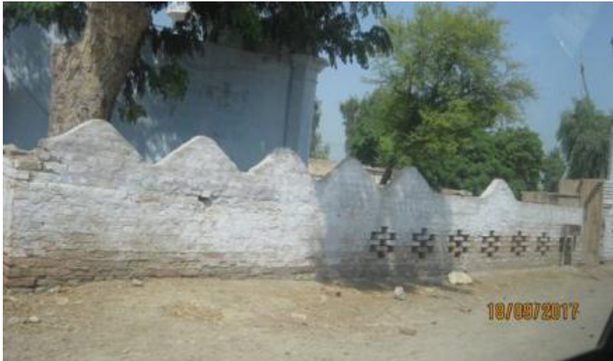
Mosque across the existing alignment at Rahim Abad Laro
