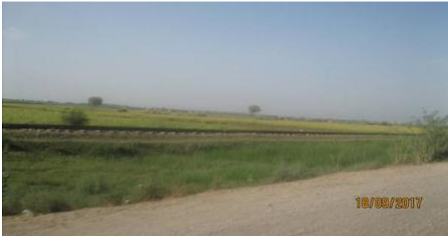
Railway track along the existing alignment around 10-15m from N-55
