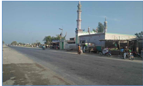
Plate 18: A view of affected mosque at Chainage 144+250 Gulanpur, Kashmir.
