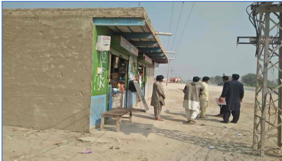
Plate 6: A view of affected structure and Electric poles at Starting point of Kandhkot – Kashmir Section near Jamia Masjid Khawaja Ghreeb Nawaz.
