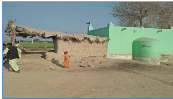
Plate 7: A view of affected mosque and thatched shed at 138+950
