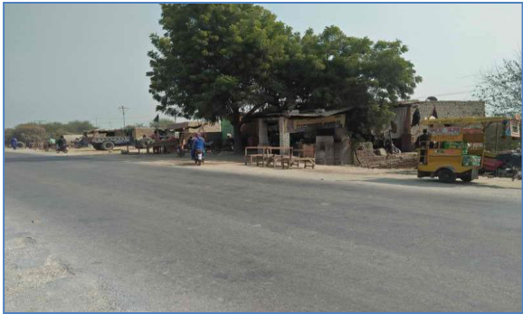
Plate 4: A view of affected structure at Goth Jahan Khan Bangwar.
