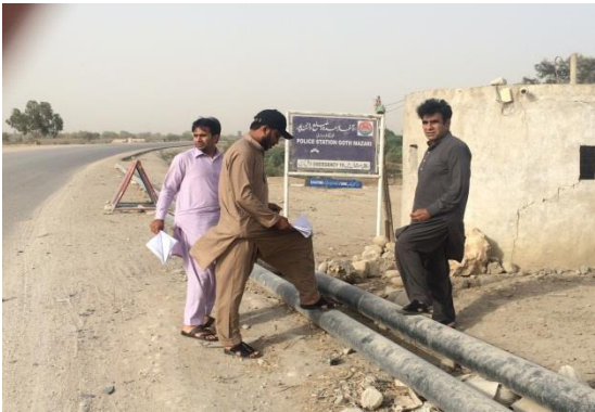
Plate 7: Road section located in the jurisdiction of Kashmor – Rajanpur road Section (Punjab).
