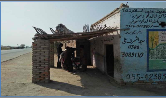
Plate 16: A view of affected structure at Machi Bindo, UC Jamal, Shikarpur
