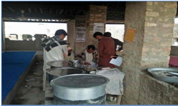
Plate 19: A view of affected structure right side at Chainage 64+535, Shikarpur
