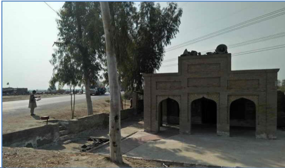
Plate 9: A view of affected mosque at Baghri Larow Shikarpur.
