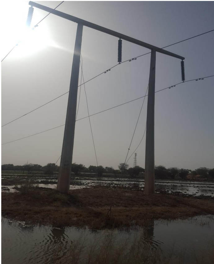
Close view of a PCC Pole erected in the agriculture productive land
