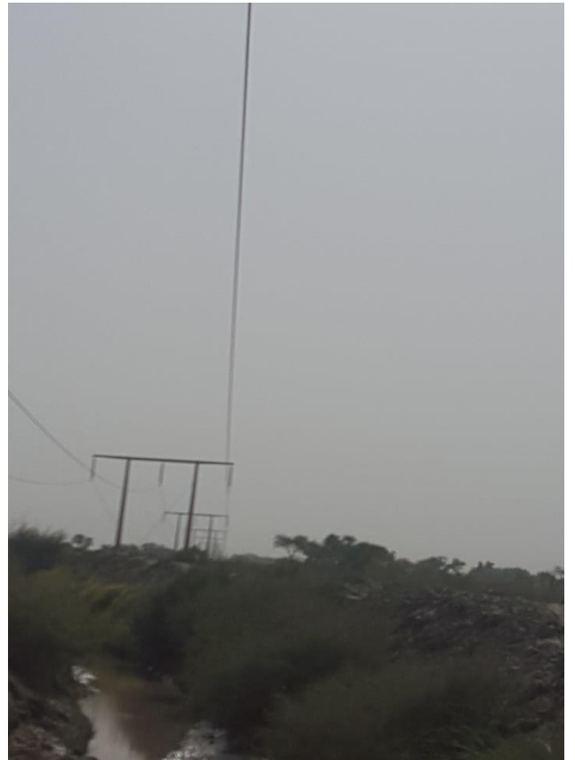
Irrigation and drainage works by the farmers kept conductors height at risk.
