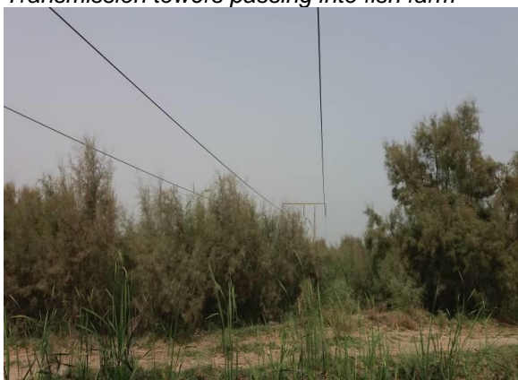
Transmission line trespassing into thickly grown bushes and trees
