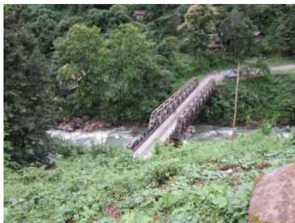
Image 3: Project road at Lokchao River Bridge in hill section
