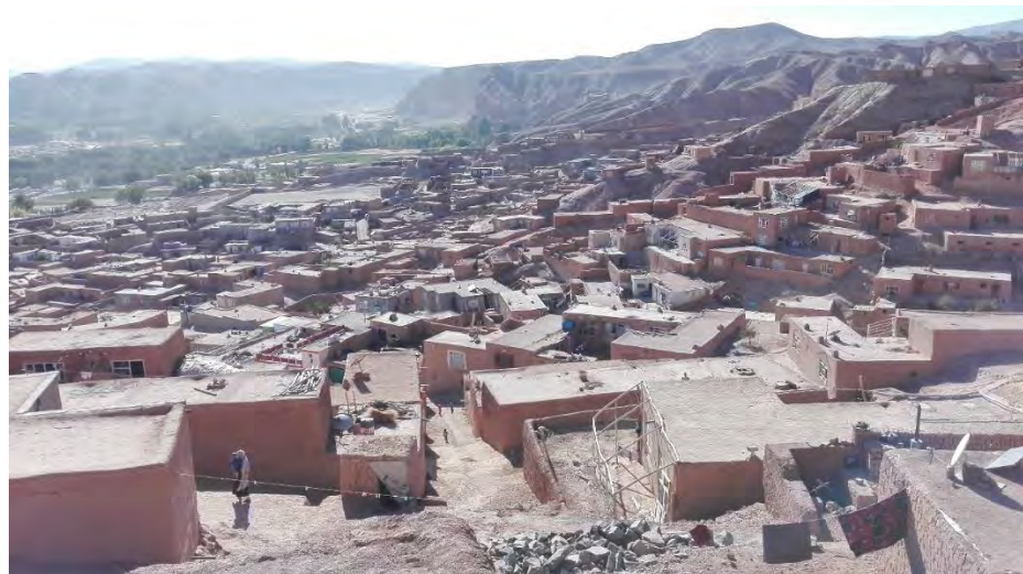
Figure 6-1: Overview of one of the villages served by the distribution network of the Haidar Abad solar power plant consisting of buried cables
