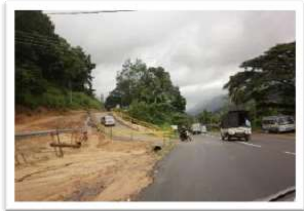
Road construction site
