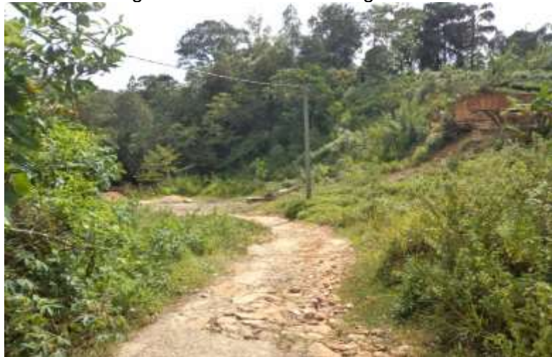
Plate 3: 2+500 - 2+600 Gravel road section
