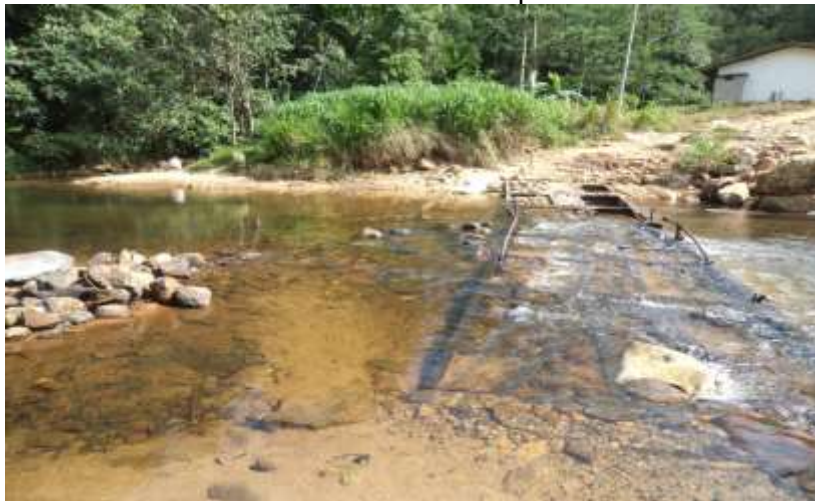
Plate 5: Road crosses Wewala Ela at 2+900 - 3+000km
