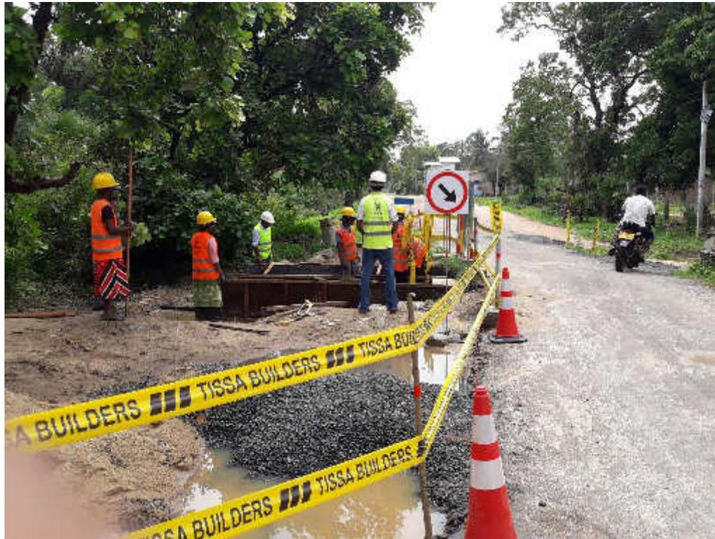
**Picture 06: – Developed safety arrangement at culvert work site – PO3 – 24.11.2016**
