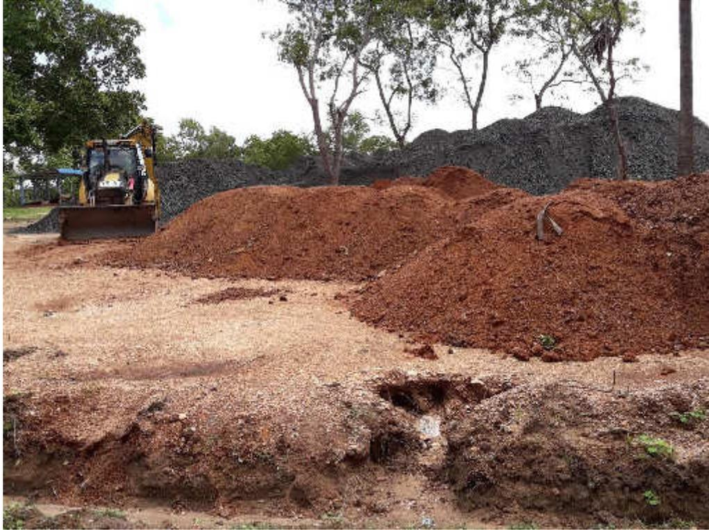
**Picture 03: – Stoked pile yard without soil erosion preventive measures – PO3-
