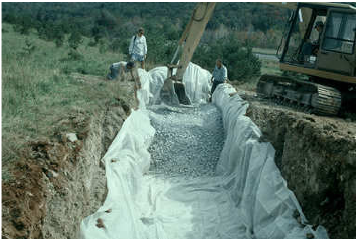
Photo 4-1: Limestone gravel being placed in lined ALD trench
