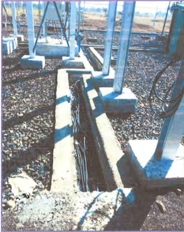
Cable Trench Line & Fencing Work at 33/11KV BIJURI S/s District Chhindwara
