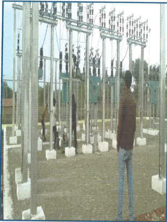
Bifurcation of 33 KV line at Pahadiya Substation, Rewa
