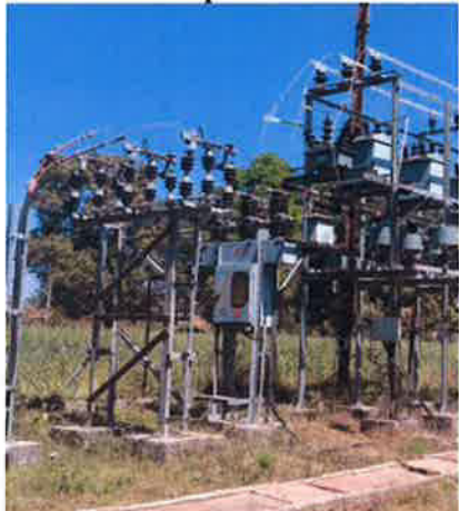
Installation of Capacitor Bank & Control Panel at Chirapatla and Public Consultation
