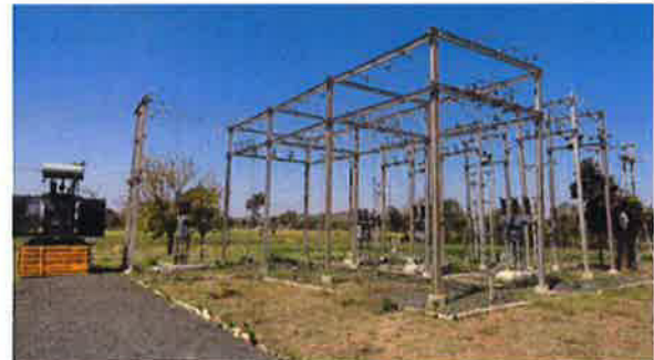
Installation of Incoming 33KV and outgoing 11 KV lines, ME & Power transformer
