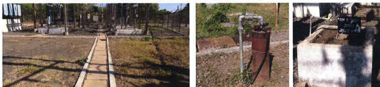
Installation of Cable Tranche, Borewell and Earthing pad
