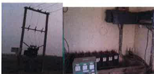
Distribution Transformer & Battery Charger
