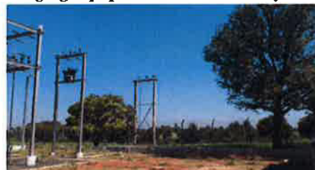
Installation of Power Transformer & connected with 11 KV & 33 KV lines
