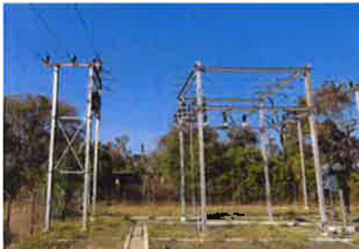
Installation of Transformer, ME and incoming 33 KV & outgoing 11 KV Lines
