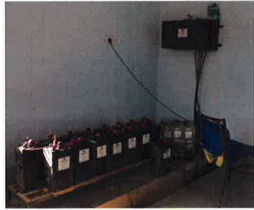
Installation of Control Panel, Battery Bank and Cable Tranche
