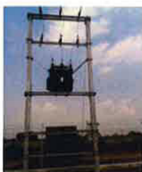
Installation of Distribution Transformer, incoming 33 , outgoing 11 KV Lines & Power Transformer
