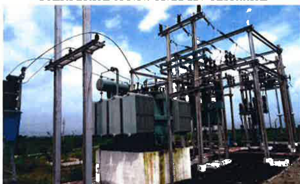
Installation of Power Transformer, 33 KV incoming & 11 KV Outgoing lines
