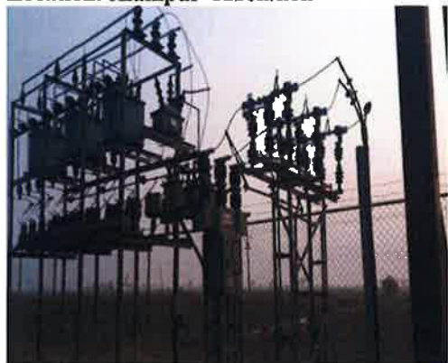
Installation of Capacitor Bank & Control Panel at Alampur Substation and Public Consultation
