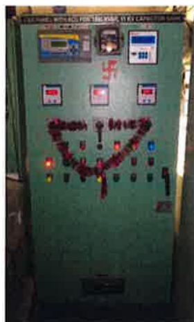
Installation of Capacitor Bank & Control Panel at Sonkachh Substation and Public Consultation
