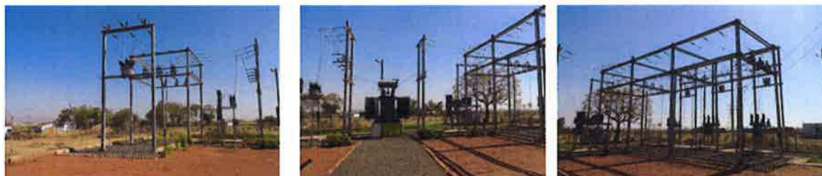
Installation of Incoming 33KV and outgoing 11 KV lines, ME & Power transformer
