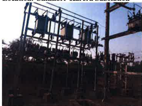
Installation of Capacitor Bank & Control Panel at Chinnori Karera and Public Consultation
