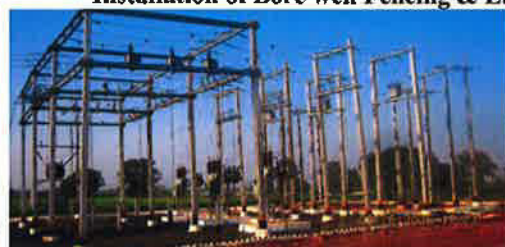
Installation of Distribution Transformer, incoming 33 , outgoing 11 KV Lines & Power Transformer
