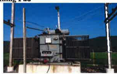
Installation of Distribution Transformer, incoming 33 , outgoing 11 KV Lines & Power Transformer
