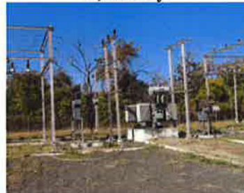
Installation of Transformer, ME and incoming 33 KV & outgoing 11 KV Lines
