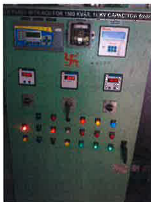
Installation of Capacitor Bank & Control Panel at Dabra Grameen and Public Consultation
