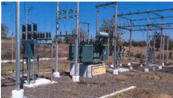
Installation of Power Transformer & connected with 11 KV line, 33 KV lines & Fire Control Facility
