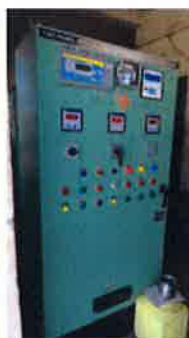
Installation of Capacitor Bank & Control Panel at Hasua Substation and Public Consultation
