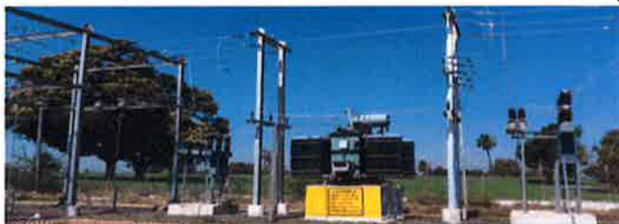
Installation of Power Transformer & connected with 11 KV & 33 KV lines
