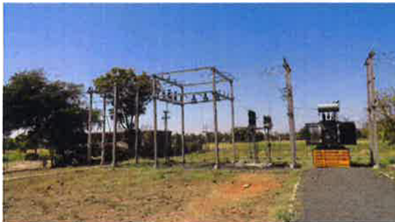
Installation of Incoming 33KV and outgoing 11 KV lines, ME & Power transformer
