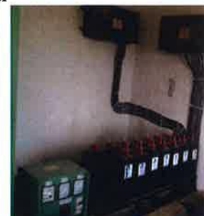
Cable Tranche, Control Panel, Battery Bank, Input-Output and Battery Charger
