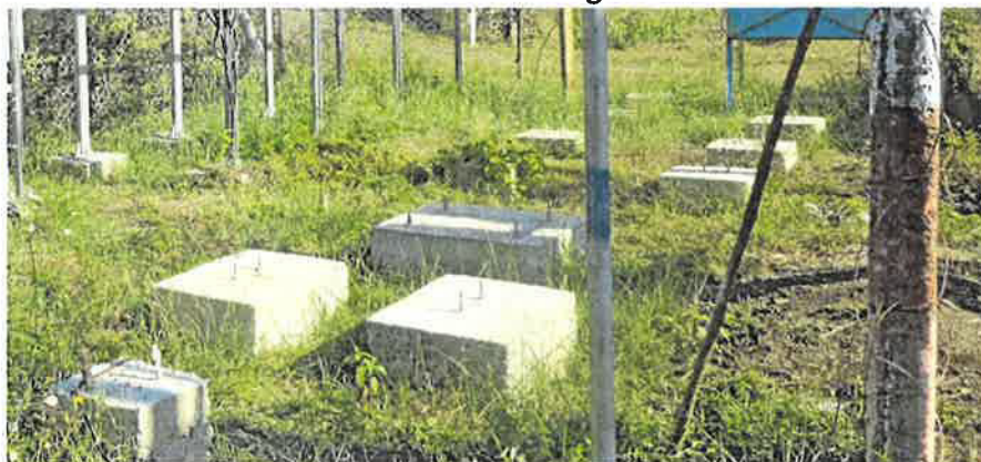
Figure 13: Construction of Foundation Pad for installation of 11 KV, 1500 KVAR Capacitor Bank at Badona substation district Gwalior
