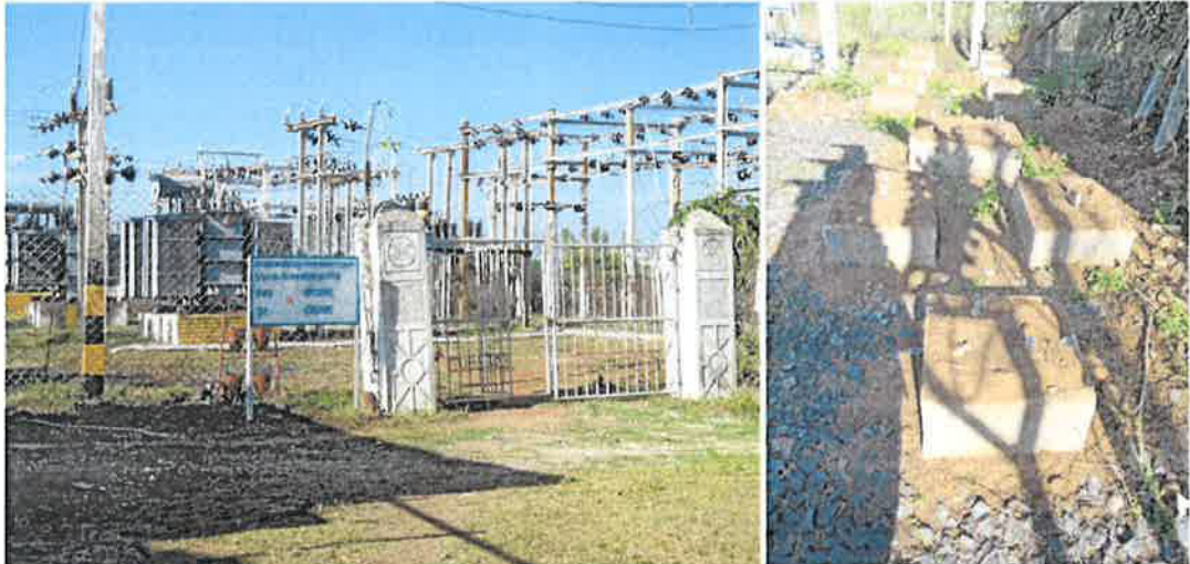
Figure 9: Construction of Foundation Pad for installation of 11 KV, 1500 KVAR Capacitor Bank at Dolariya substation district Hoshangabad
