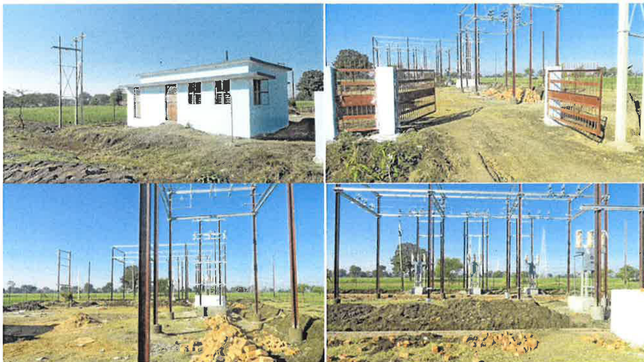
Figure 3: Construction of New 33/11 KV Substations at Dabri village district Sehore
