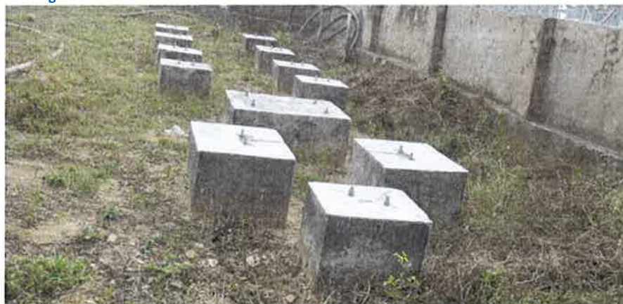
Figure 15: Construction of Foundation Pad for installation of 11 KV, 1500 KVAR Capacitor Bank at Banmore substation district Morena
