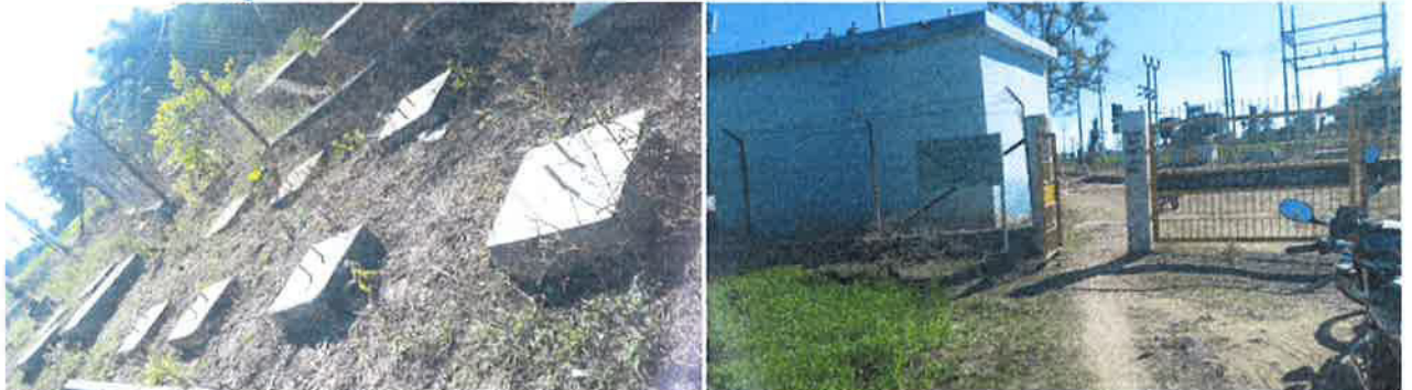
Figure 11: Construction of Foundation Pad for installation of 11 KV, 1500 KVAR Capacitor Bank at Bhadus substation district Betul
