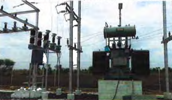
Installation of Transformer, 11 KV Feeders & ME
