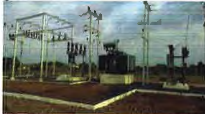
Installation of incoming 33 KV Lines, Transformer, Feeder and outgoing 11 KV Lines
