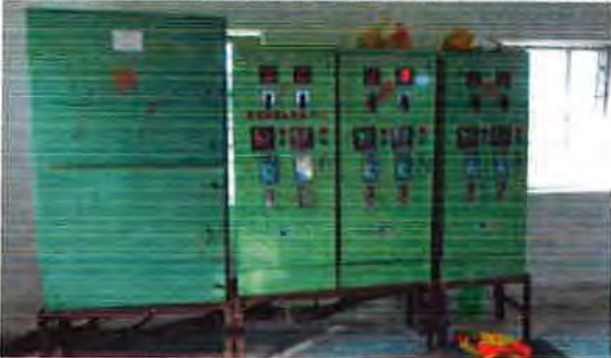
Installation of Control Panels & Feeders, ME and Bus bar
