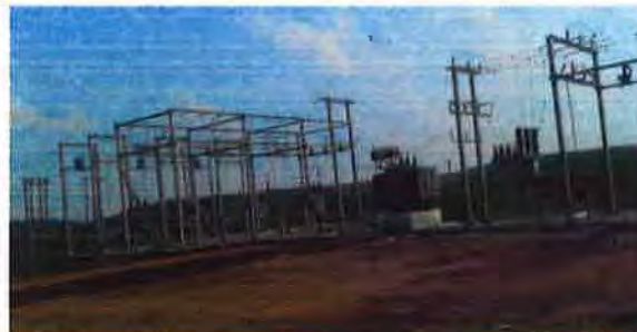
Installation of Distribution Transformer, ME, incoming 33 & outgoing 11 KV Lines
