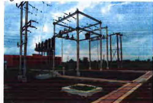
Installation of Fencing, Earth work, Earthing Pad, 33 & 11 KV Feeders, ME and incoming & Outgoing lines
