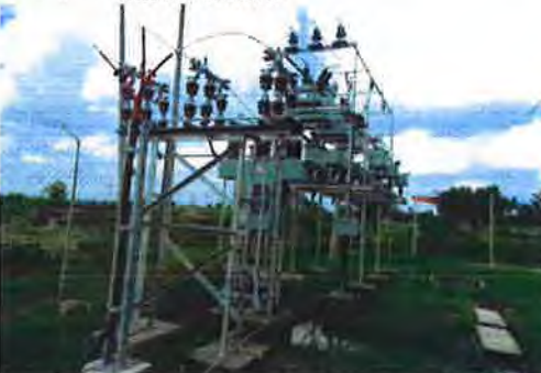
Installation of Capacitor Bank & Control Panel at Shrine Board Substation
