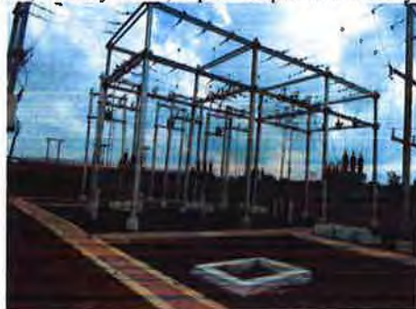
Installation of Fencing, Earth work, Earthing Pad, 33 & 11 KV Feeders, ME and incoming & Outgoing lines
