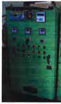
Installation of Capacitor Bank & Control Panel at Shrine Board Substation
