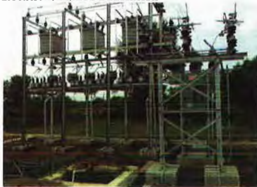
Installation of Capacitor Bank & Control Panel at Kaned Substation and Public Consultation
