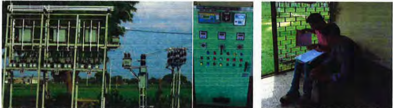
Installation of Capacitor Bank & Control Panel at Kachnow Kalan Substation and Consultation with DISCOM-C Staff
