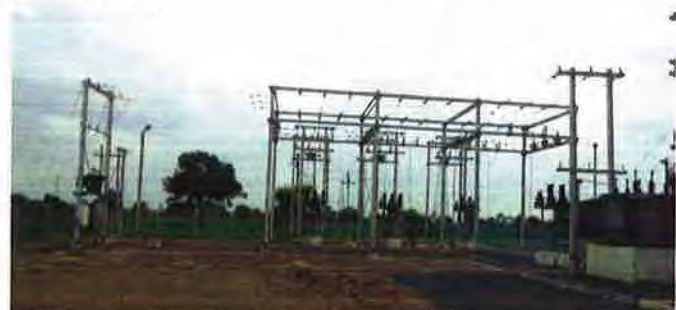
Installation of incoming 33 KV ME & Lines, Transformer, Feeder and outgoing 11 KV Lines
