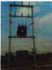
Installation of Distribution Transformer, ME, incoming 33 & outgoing 11 KV Lines
