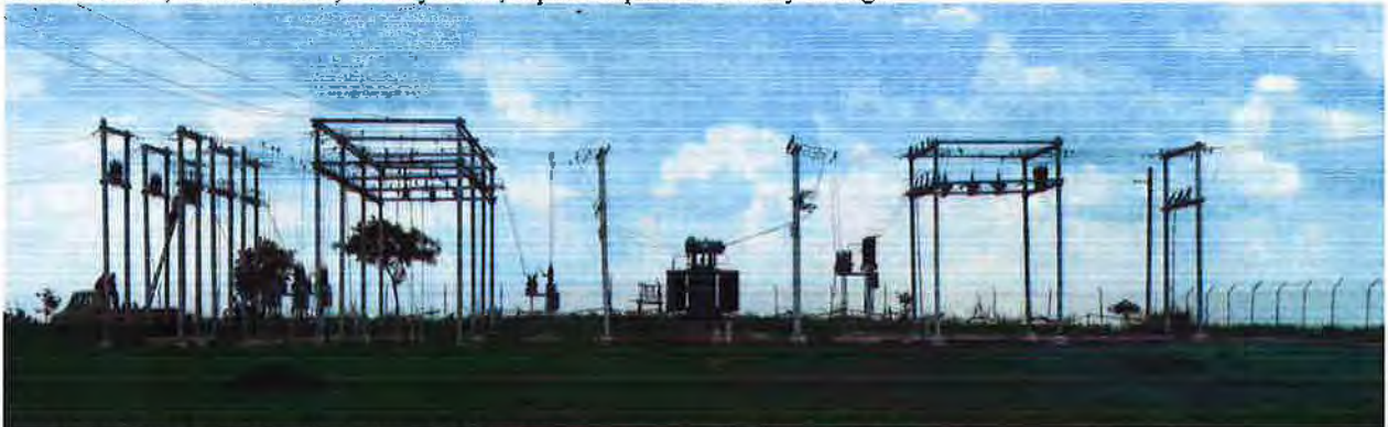
Installation of Distribution Transformer, ME, incoming 33 & outgoing 11 KV Lines
