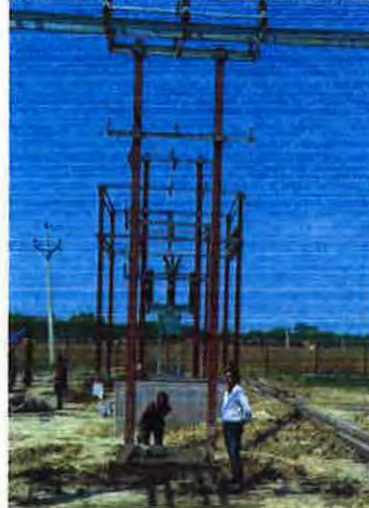
Installation of 33 KV ME, Construction of Foundation pad for Transformer and Cable Tranche
