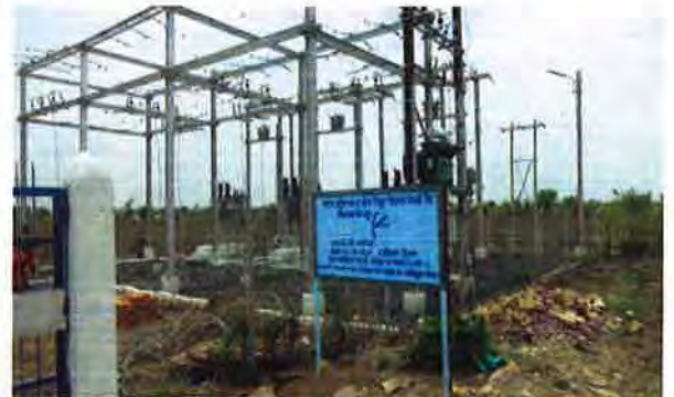
Installation of incoming 33 KV Lines, 11 KV Feeder, ME, Distribution Transformer and outgoing 11 KV Lines
