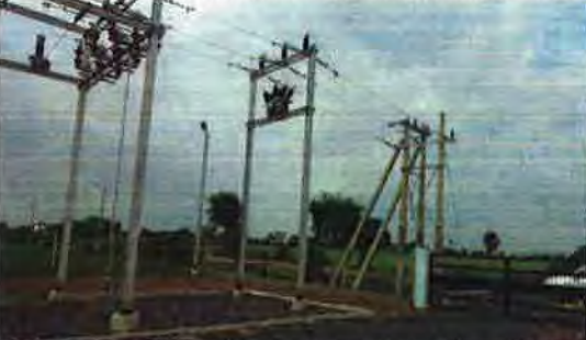
Installation of incoming 33 KV ME & Lines, Transformer, Feeder and outgoing 11 KV Lines
