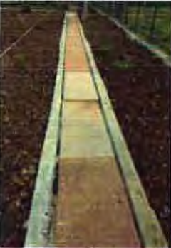
Cable Tranche & Earthing Pad & Fencing
