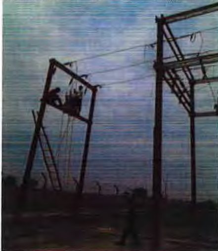
Installation of 33 KV ME, Construction of Foundation pad for Transformer and Cable Tranche
