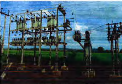
Installation of 1500 KVAR Capacitor Bank and Control panel at Jamani Substation and Public Consultation
