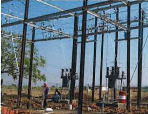
Installation of 11 KV Feeders, 33KV Feeder, ME & Power transformer is under progress
