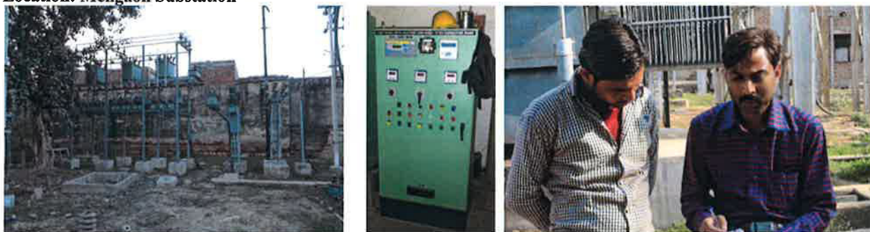
Installation of Capacitor Bank & Control Panel at Mehgaon Substation and Consultation with DISCOM-C Staff
