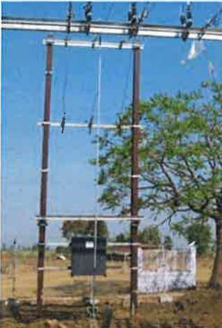
Installation of Distribution transformer and construction of earthing pad is under progress
