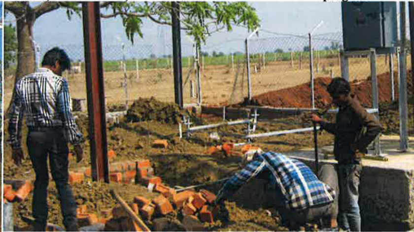
Installation of Distribution transformer and construction of earthing pad is under progress
