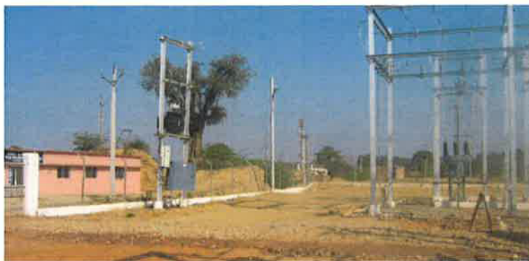
Installation of Control Panel, Distribution transformer & fencing
