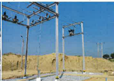
Installation of Power Transformer, incoming 33 KV and outgoing 11 KV Lines
