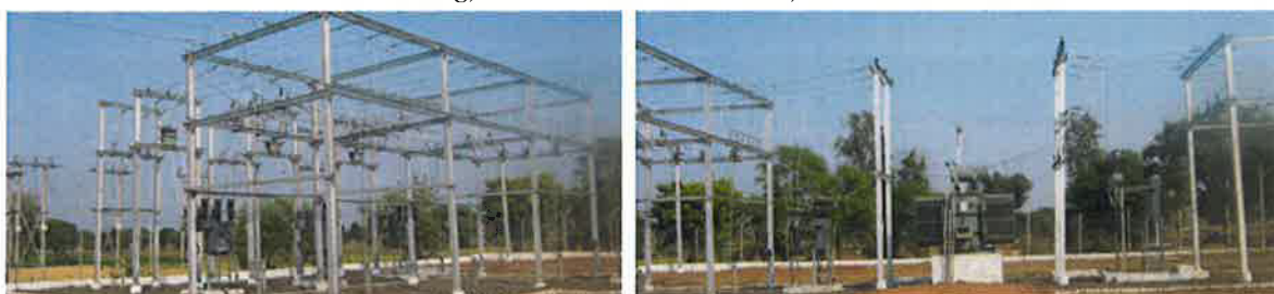
Installation of 11 KV Feeders, 33 KV Feeder, Power Transformer & ME
