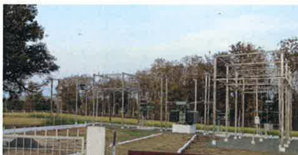
Installation of 33 & 11 KV Feeder and incoming and outgoing lines
