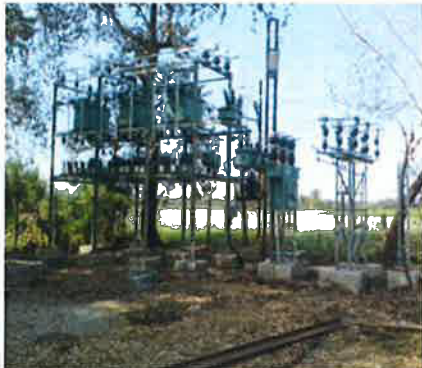
Installation of Capacitor Bank & Control Panel at Chachoda Substation and Public Consultation
