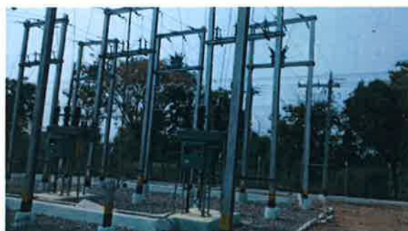
Installation of 11 KV feeders
