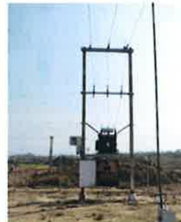
Installation of Bore well, 33 KV and 11 KV Feeder, ME and Distribution Transformer
