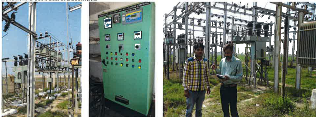
Installation of Capacitor Bank & Control Panel at Dabra Rural Substation and Public Consultation
