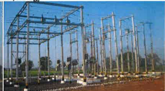
Installation of 33 KV and 11 KV Feeder, ME and Power transformer
