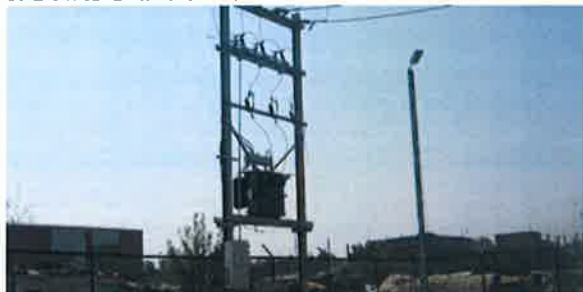
Installation of 11 KV Feeders & Distribution Transformer
