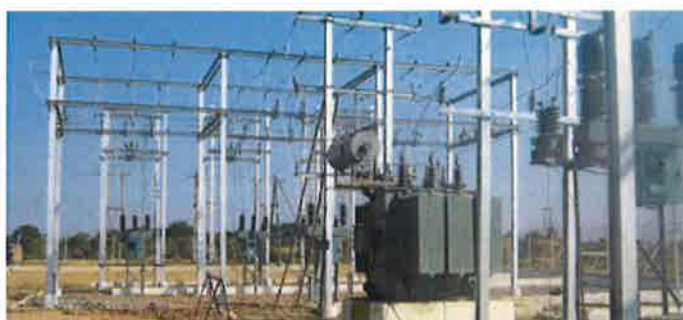
Installation of Power Transformer, 11 KV Feeders and cable tranche
