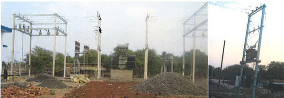
Installation of Power Transformer, ME, 33 KV Feeder and Distribution transformer
