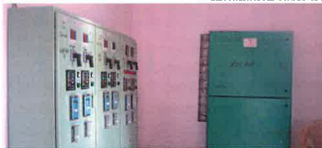
Installation of Control Panel & Power Transformer
