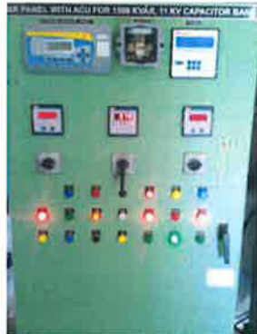
Installation of Capacitor Bank & Control Panel at Chachoda Substation and Public Consultation
