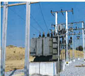
Installation of Power Transformer, incoming 33 KV and outgoing 11 KV Lines
