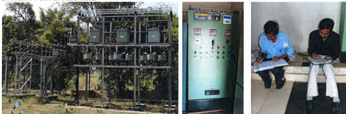
Installation of Capacitor Bank & Control Panel at Bhadus Substation
