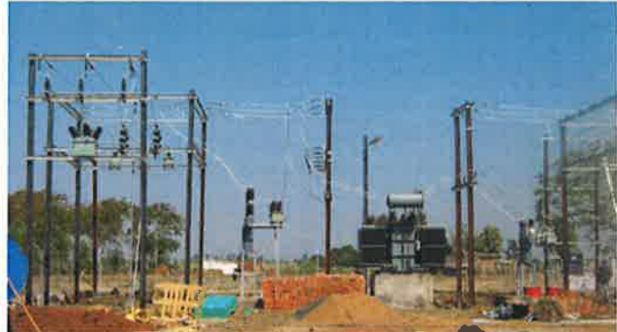
Installation of 11 KV Feeders, 33KV Feeder, ME & Power transformer is under progress
