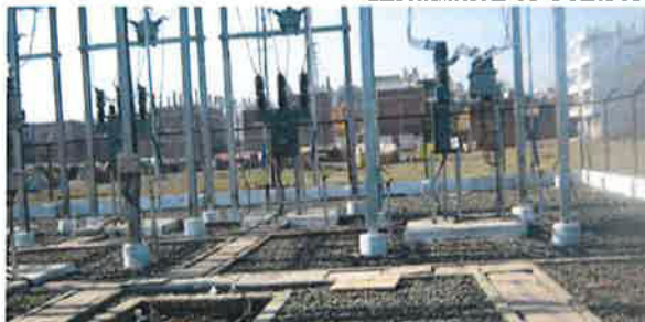
Installation of 11 KV Feeders & Distribution Transformer
