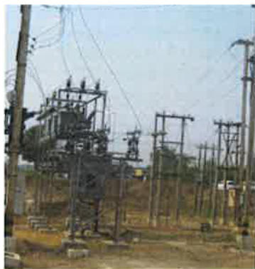
Installation of Capacitor Bank & Control Panel at Kotighar Substation and Public Consultation
