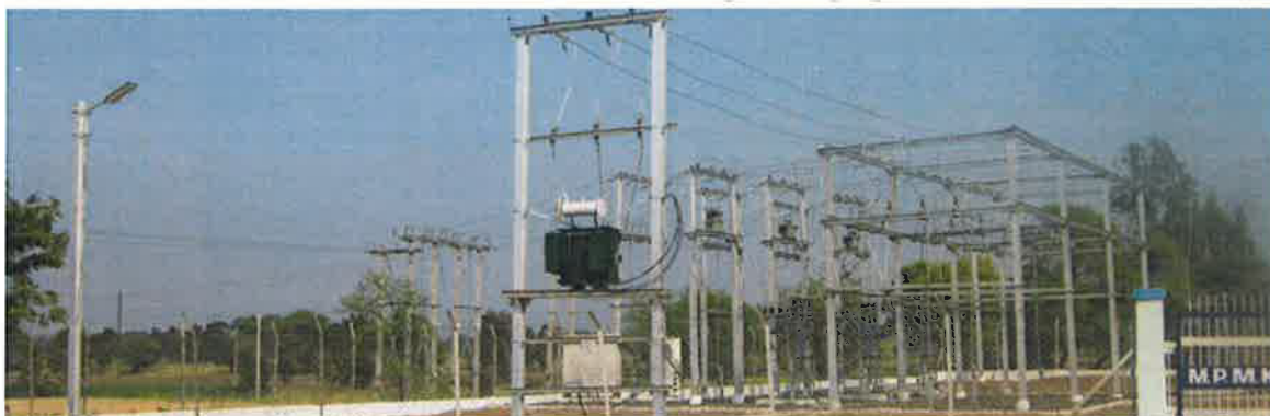
Installation of fencing, Distribution Transformer, 11 KV Feeders & ME
