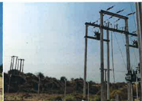
Installation of Power Transformer, incoming 33 KV and outgoing 11 KV Lines
