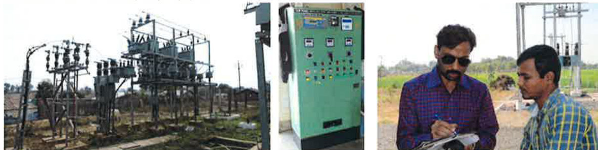
Installation of 1500 KVAR Capacitor Bank & Control panel at Semri Harchand Substation and Public Consultation
