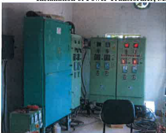
Installation of Control Panel and 11 KV Feeders & ME
