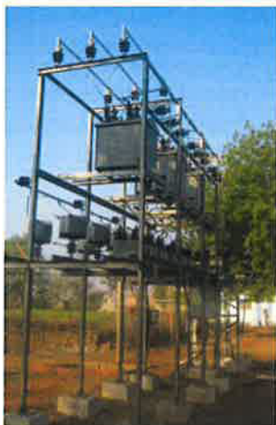
Installation of Capacitor Bank & Control Panel at Pohari Substation and Public Consultation
