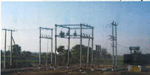
Installation of 33 KV and 11 KV Feeder, ME and Power transformer
