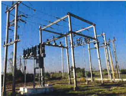
Installation of Incoming 33KV and outgoing 11 KV lines, ME & Power transformer
