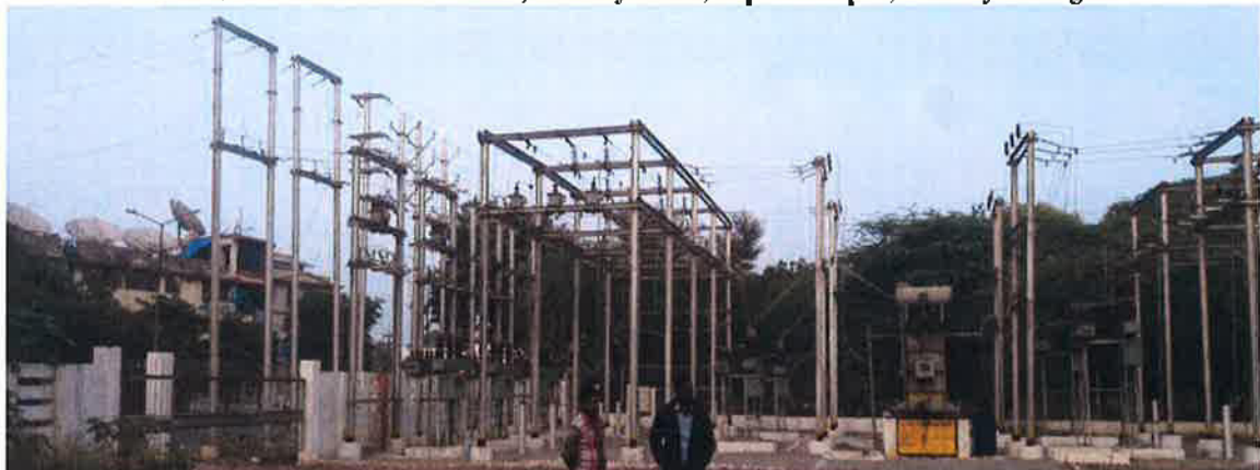
Installation of Transformer and Installation of ME, incoming 33 KV & outgoing 11 KV Lines
