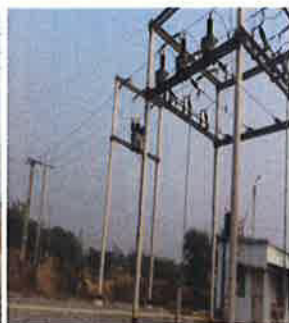
Installation of Power Transformer, incoming 33 KV , outgoing 11 KV Lines & Distrubution Transformer
