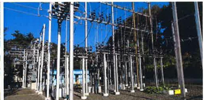
Installation of Transformer, 33 & 11 KV Feeder, ME and incoming and outgoing lines
