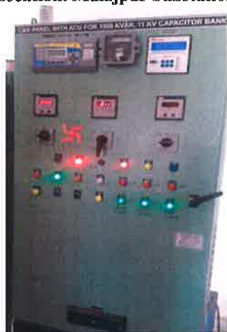
Installation of Capacitor Bank & Control Panel at Malajpur Substation
