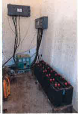
Installation of Signage Board, Contol Panel, Battery bank and Meter box
