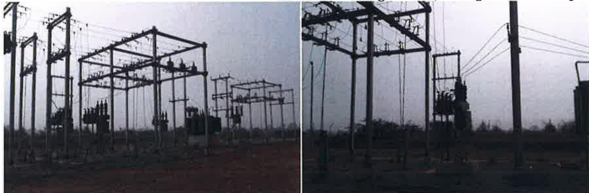
Installation of Power transformer, incoming 33 KV , outgoing 11 KV Lines
