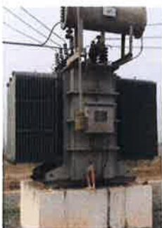
Installation of Power Transformer, incoming 33 KV , outgoing 11 KV Lines & Distrubution Transformer
