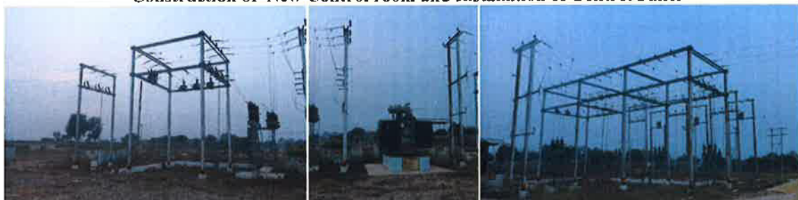
Installation of Power Transformer, 33/11 KV lines, ME and Feeders
