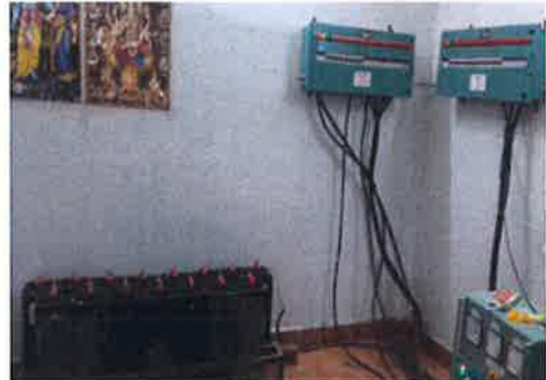
Installation of Control Panel, Battery Bank, Input-Output, Battery Charger
