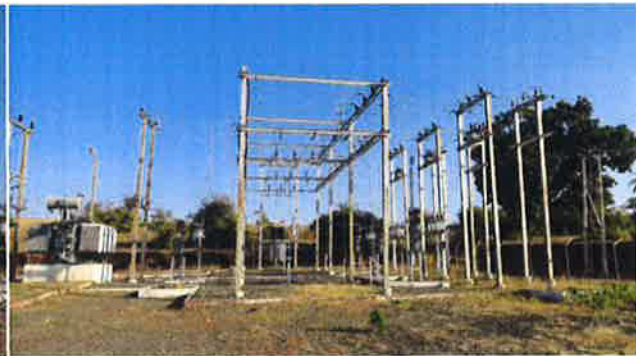
Installation of Transformer, ME and incoming 33 KV & outgoing 11 KV Lines
