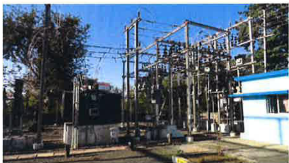
Installation of Transformer, 33 & 11 KV Feeder, ME and incoming and outgoing lines
