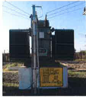
Installation of Incoming 33KV and outgoing 11 KV lines, ME & Power transformer
