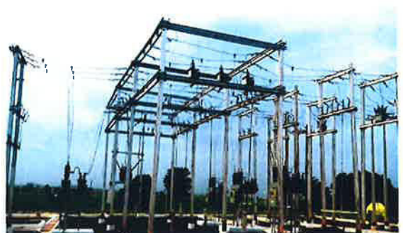
Installation of 33 & 11 KV Feeder and incoming and outgoing lines
