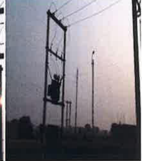
Installation of Power Transformer, incoming 33 KV , outgoing 11 KV Lines & Distrubution Transformer
