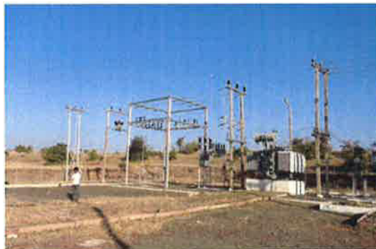
Installation of Transformer, ME and incoming 33 KV & outgoing 11 KV Lines
