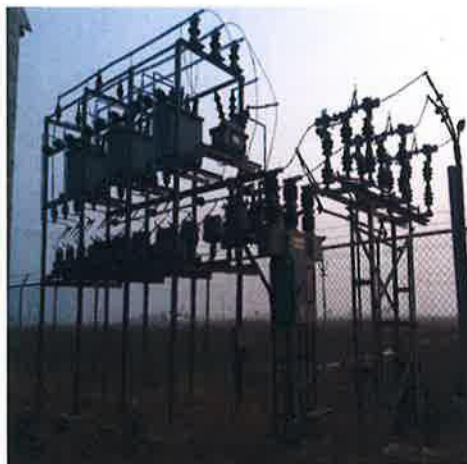
Installation of Capacitor Bank & Control Panel at Malajpur Substation
