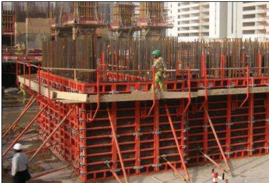
Photo 5: A typical picture of a steel reinforcing for building foundations and small structural columns
